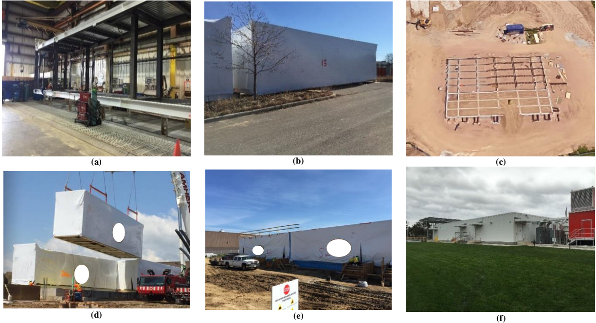
Figure 5.2. The case study during: (a) fabrication and assembly processes, (b) temporary storage area, (c) site preparation and building concrete foundation, (d) modules installation at project site, (e) connection of MEP systems, and (f) completed building.
