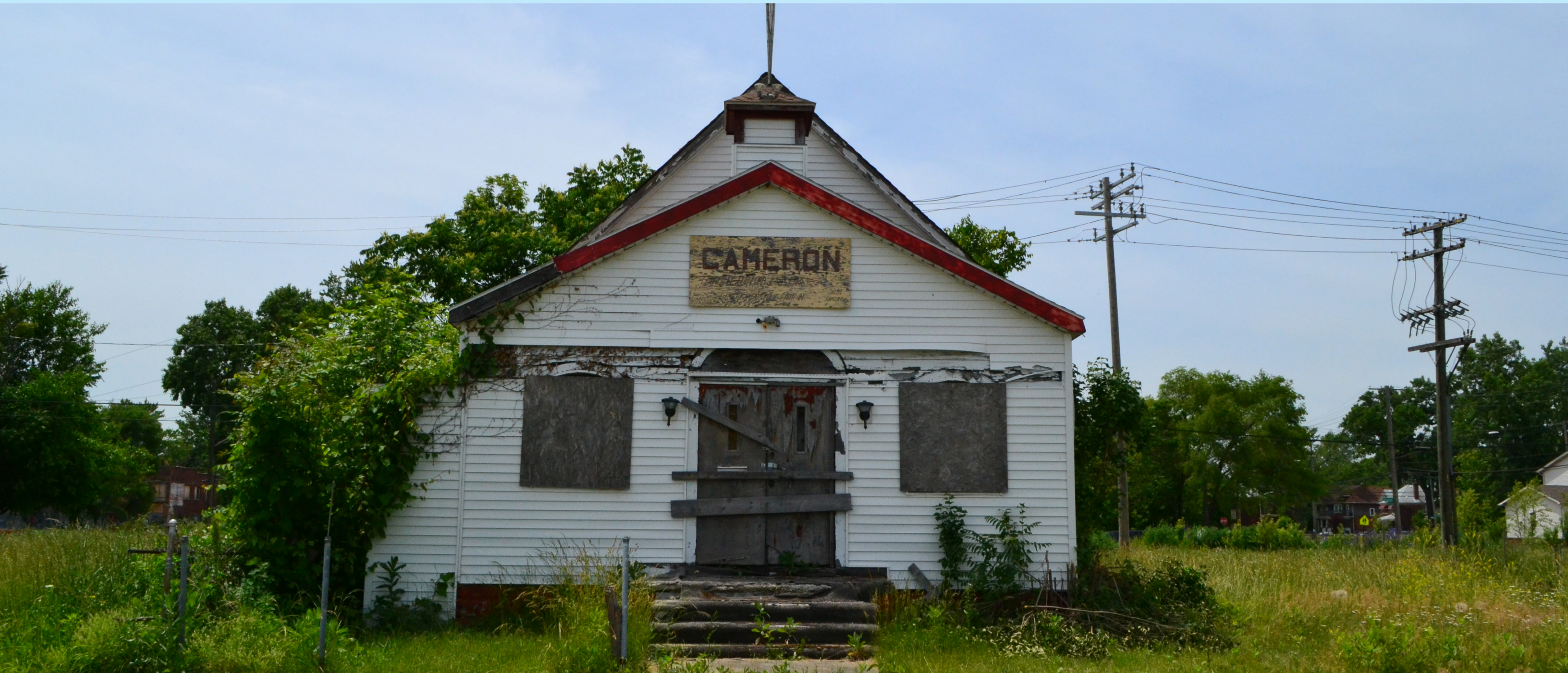
Fig 3.14 Dilapidated Church, Detroit 2018
