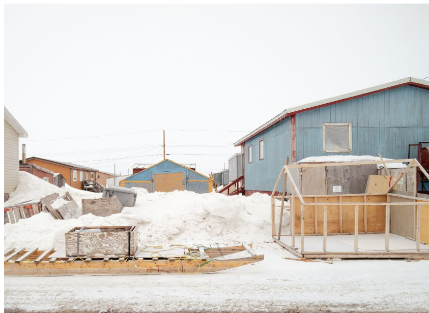
f 2.47 A modified Weber house, with a tent frame under construction in the foreground, storage shed in the back left and an added wind porch outside of the existing cold porch in early May, 2018.
