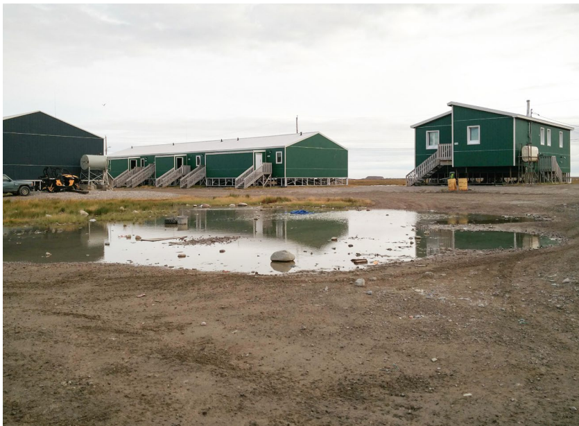
f 2.40 Land development and housing projects impose stability on the ground. However, the shifting permafrost asserts itself on buildings through the layers of fill and substructures.
