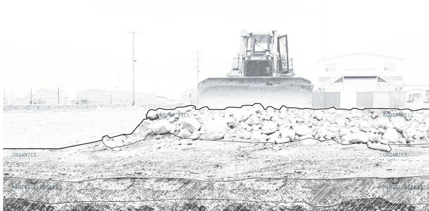
Land development over the wetlands and muskeg of arviat is enabled by a technique of artificial fill which is layered continuously over the landscape. 1-1.5 metres of rough fill is spread across the ground.
