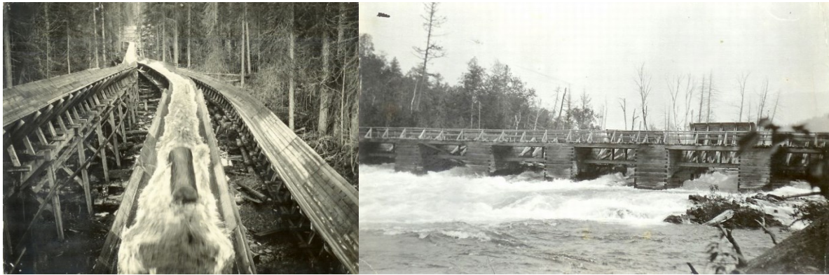
Figure 10. Left: Brennan Creek Flume; Right: Lower Adams River splash dam (Chase and District Museum and Archives Society, credit for left image to Walter F. Montgomery).
