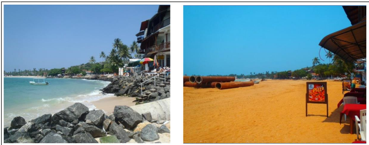
Figure 6.7: Before and after beach nourishment of Unawatuna Bay (East)
