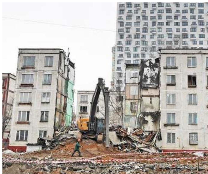
Figure 58: Demolition and reconstruction of 5,000 5-storey khrushchevka buildings in Moscow
