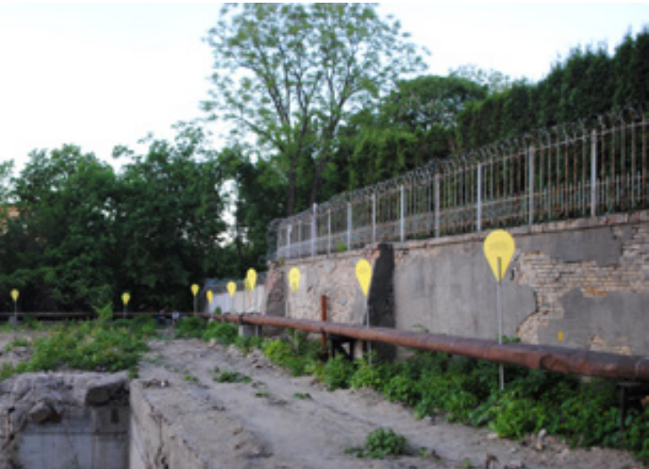
EXISTING SITE - VIEW 2
