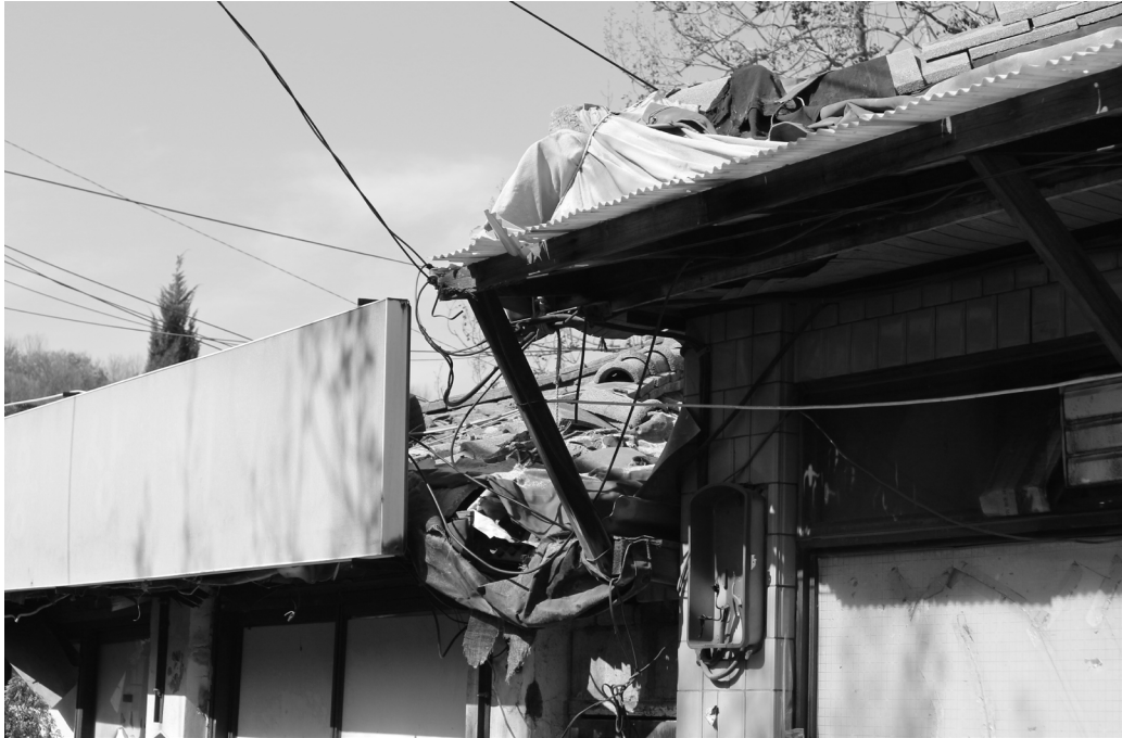
Figure 8 Roof Support for a Retail Building
