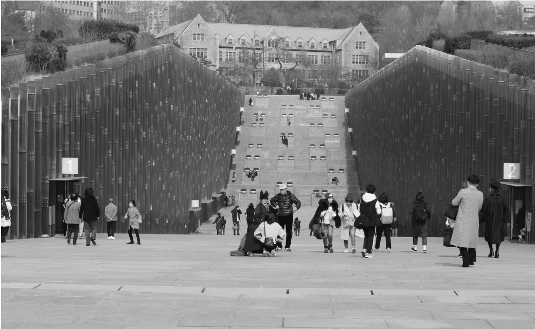
Figure 53 Ewha Womens University uses the topography to carve a valley like walkway
