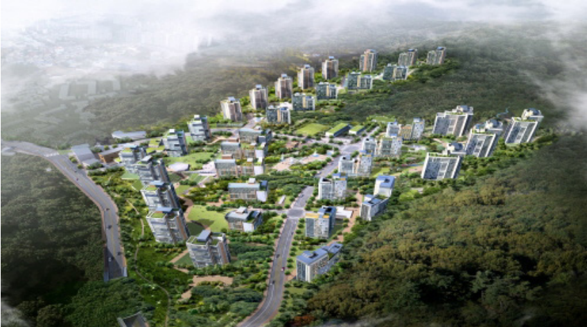
Figure 12 Proposal from 2008 from the Land and Housing Corporation to Redevelop Baeksa Village
