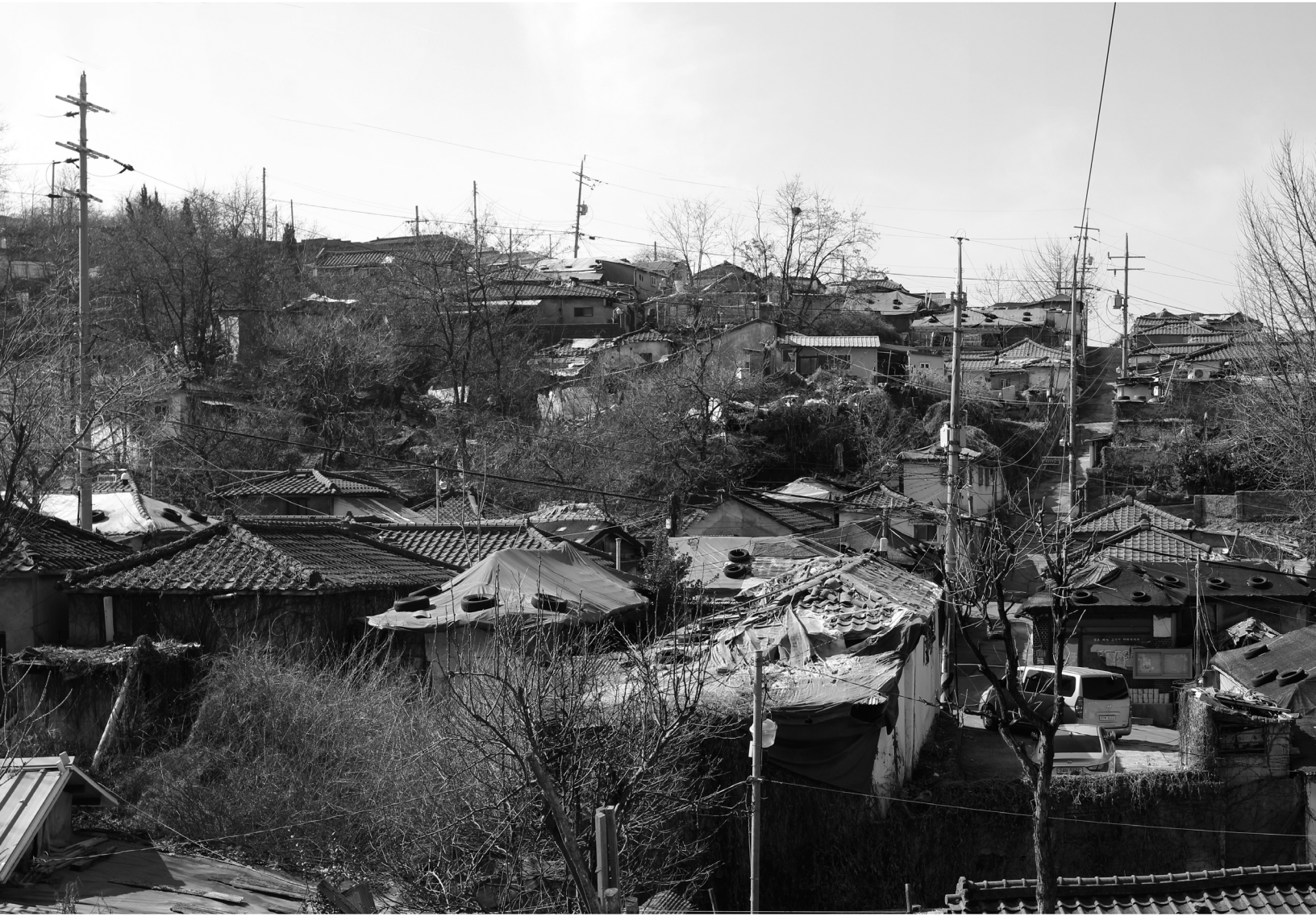
Figure 1 An Aerial View of Baeksa Village
