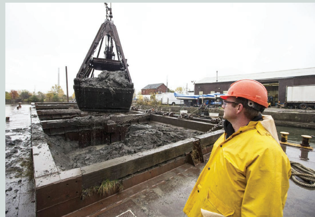
fig. 2.15 (left) dredge material dredged from the Keating Channel
