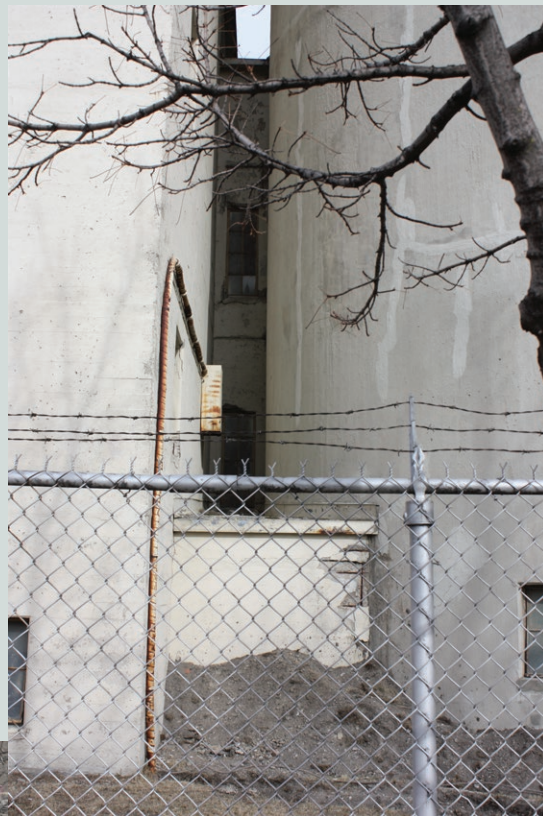
fig. 1.68 (right) Close up of Lafarge cement silos, the walls constructed of thick poured in place reinforced concrete
