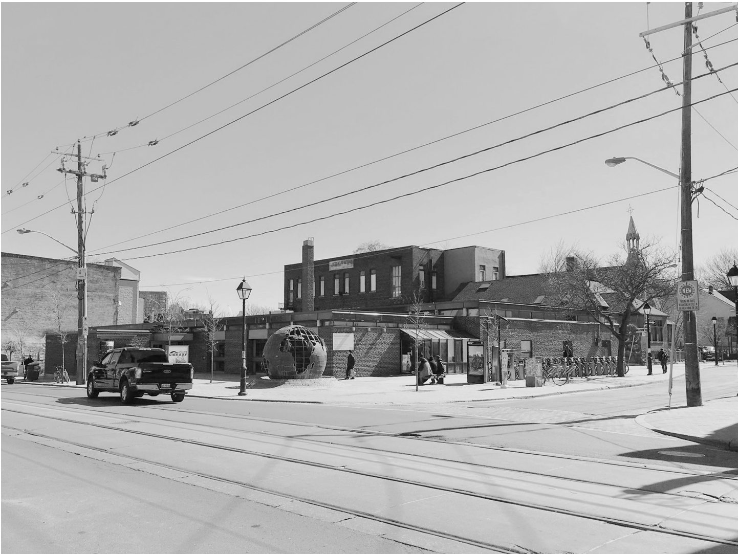
^ fig. 18 Corner view of existing Parkdale Public Library. > fig. 19 Existing Parkdale Public Library's ground floor plan.
