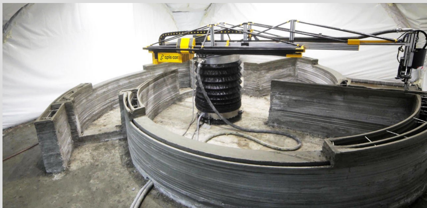
Figure 01.47 • Apis Cor Construction Image
