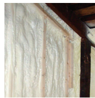
Figure 02.33 • Polyurethane Spray foam insulation, can be applied continuously as a spray, expands and hardens as it cures. Thermal, environmental, and structural performance depends on the cell size and volume.
