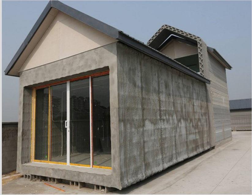
Figure 01.41 • Printed Structure
