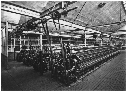
Figure 03.5 • Line Shaft A line shaft would transfer the mechanical energy from a turbine or engine and drive the factory equipment.
