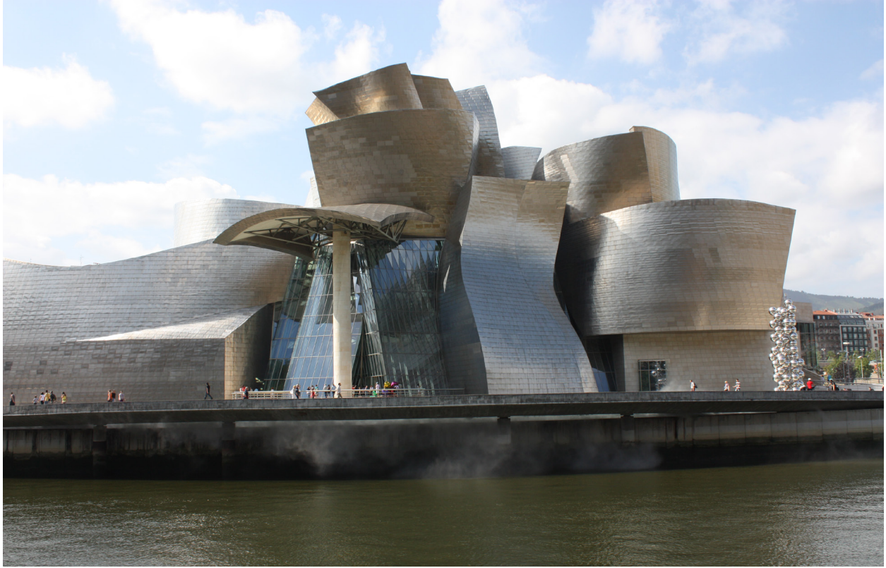
Figure 05.5 • Guggenheim Bilbao - Gehry: Complexity
