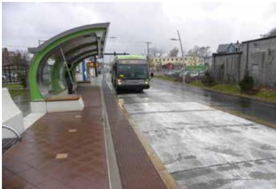
Figure 2-1. Connecticut HMA bus pad rehabilitation (Tayabji & Tyson, 2017)
