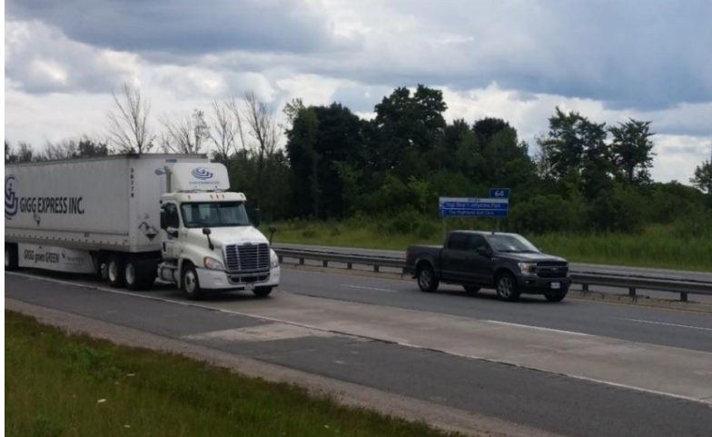
Figure 1-1. Precast concrete inlay panels installation in-service on Highway 400
