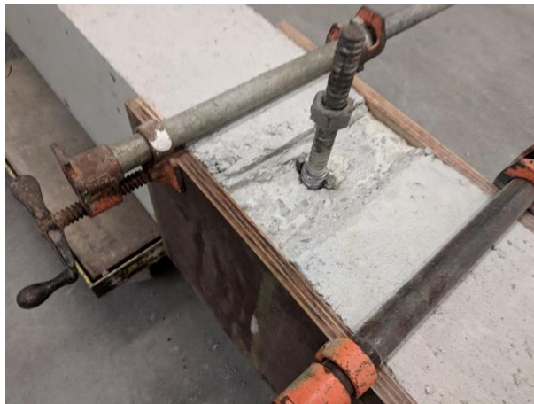
Figure 3.7 – Missing compressive concrete in BM 4.5-N
