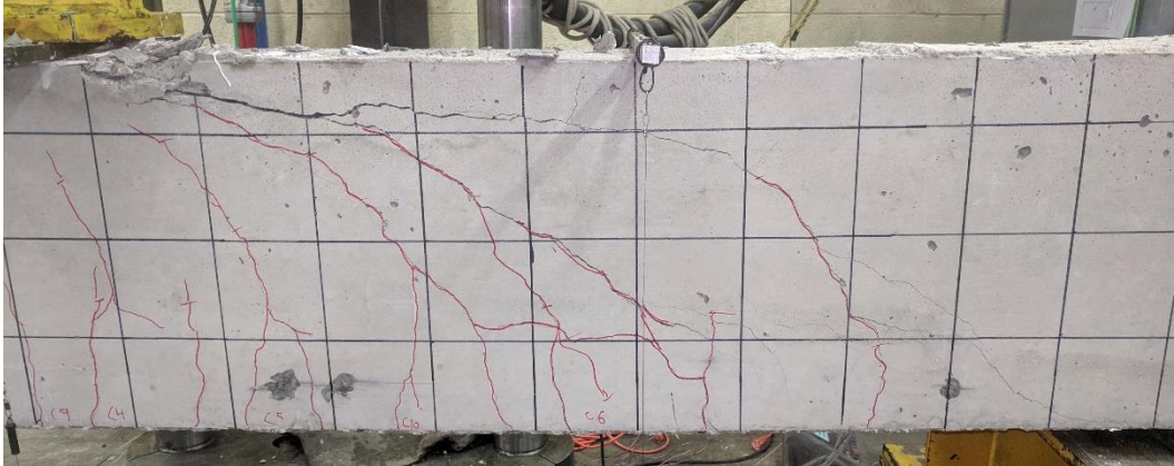
Figure 4.11 – BM 4.5-150: Crack patterns at failure
