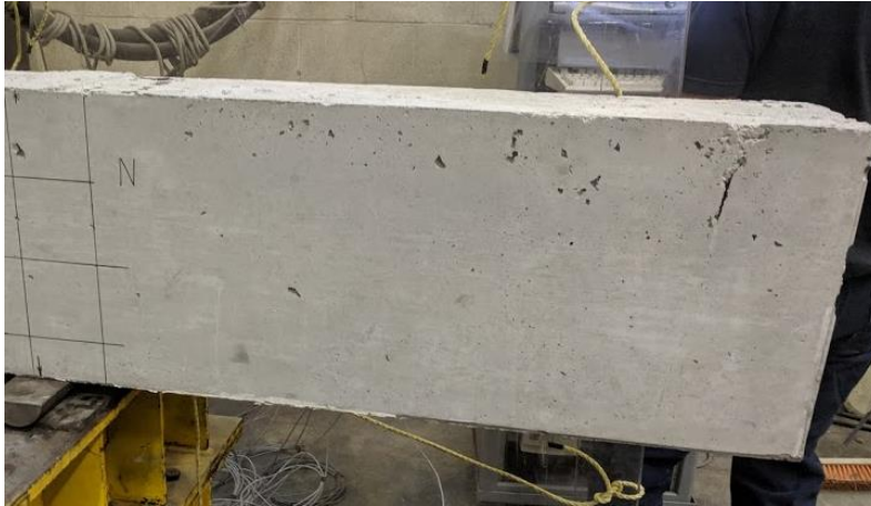
Figure 3.6 – Areas of localized cavities due to lack of consolidation in BM 4.5-N
