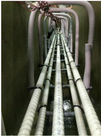
Figure 3.4 – GFRP cage in formwork with instrumentation
