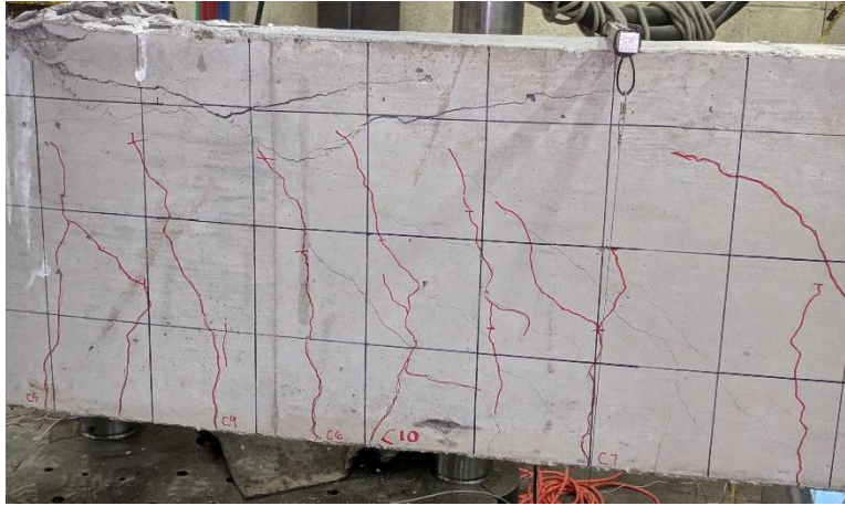
Figure 4.6 – BM 4.5-90: Crack patterns at failure
