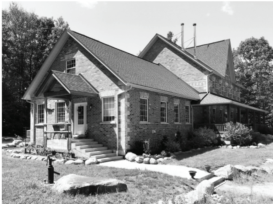
Fig 1.05 Exterior of two-storey brick house
