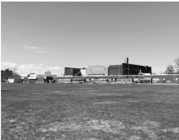
Fig 3.22 South view of school
