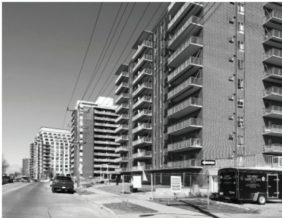
Fig 3.07 Downtown high-rise apartments
