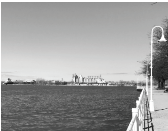
Fig 3.09 Port of Sarnia
