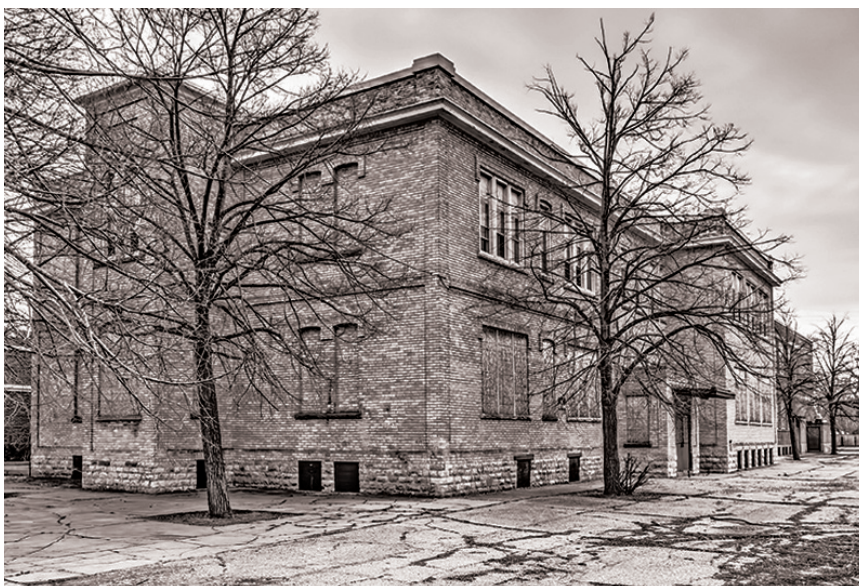
Fig 3.26 Abandoned Devine Street School
