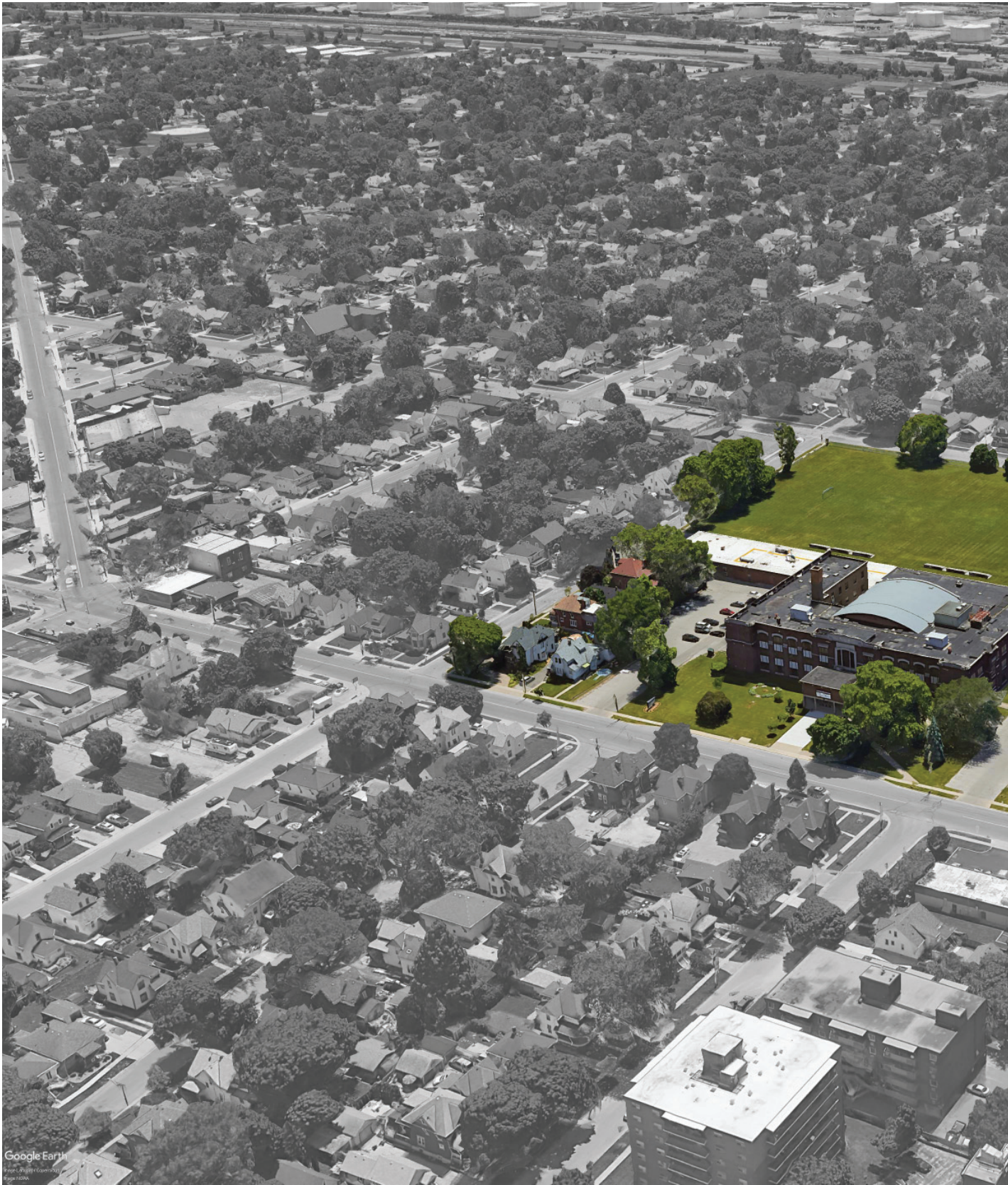
Fig 3.24 SCITS Aerial site image
