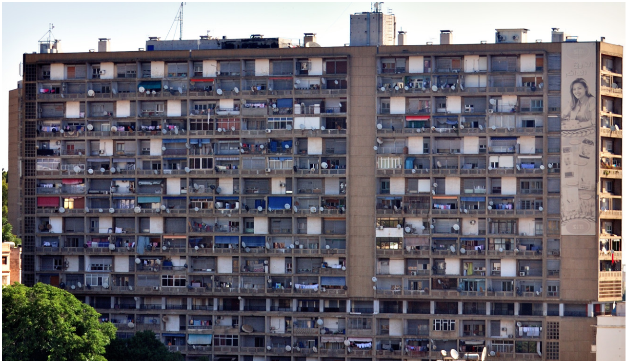
Figure 8.5 Southwest view of Aéro-Habitat
