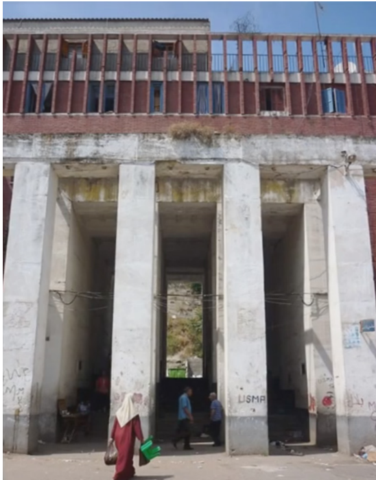
Figure 8.11 View of inner colonnade with additions
