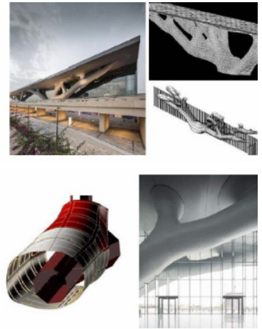
Figure 2-5: Images Qatar National Convention Centre in Doha. Clockwise descriptions: Exterior view, topology optimization output model, axonometric view of the structure, framing and cladding strategy, view of branching support.
