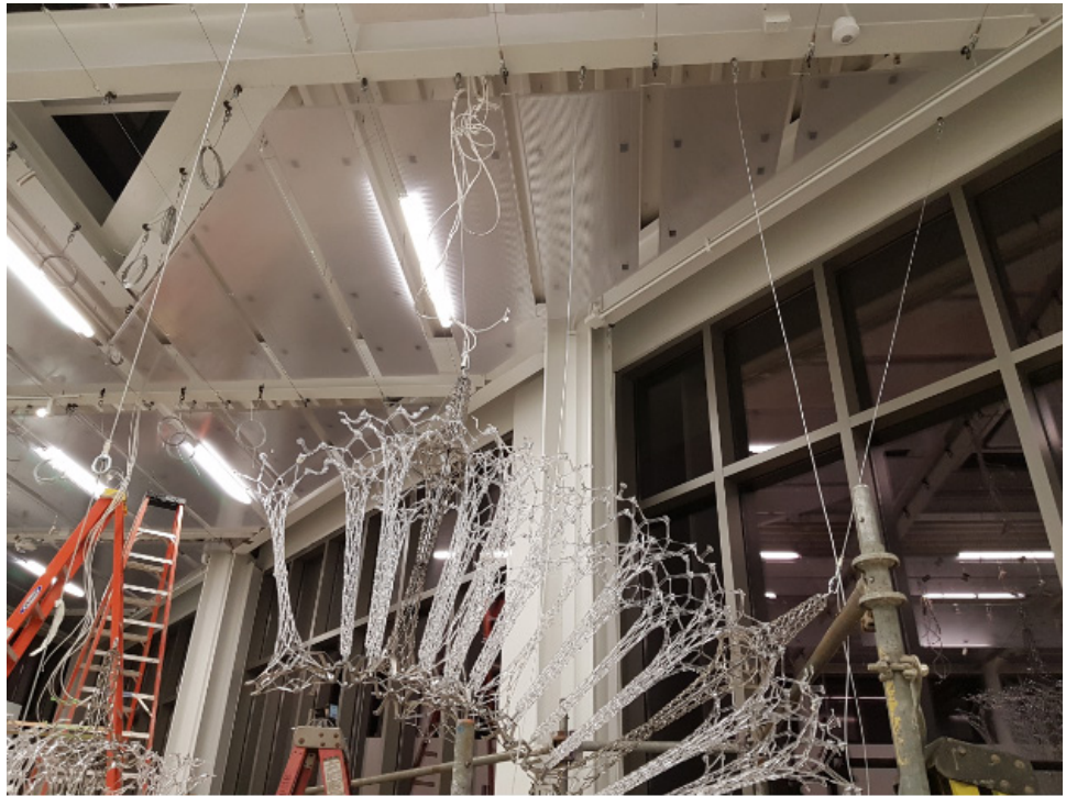
Figure 4-13: Image of the installation progress showing the angled cables.
