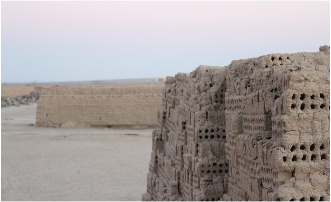
Figure 79 Unfired brick storage around the kiln
