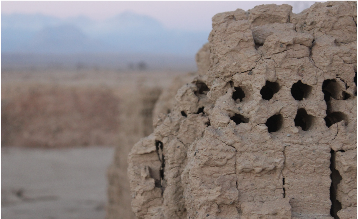
Figure 77 Unfired brick storage around the kiln
