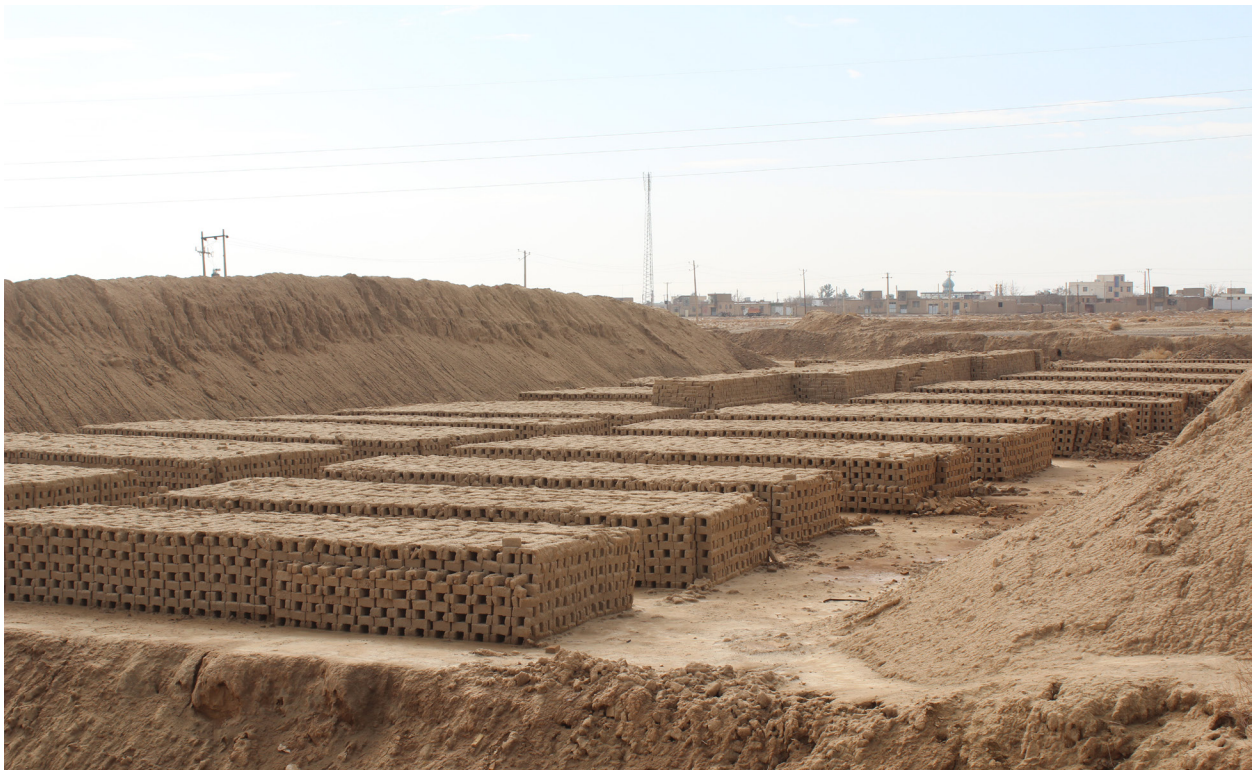
Figure 84 Unfired brick storage around the kiln
