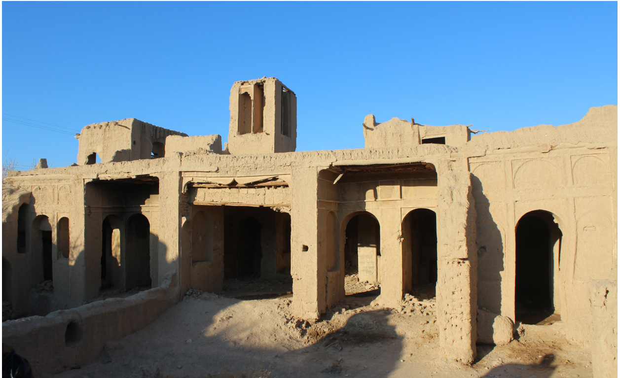
Figure 57 Abandoned house in Jazan
