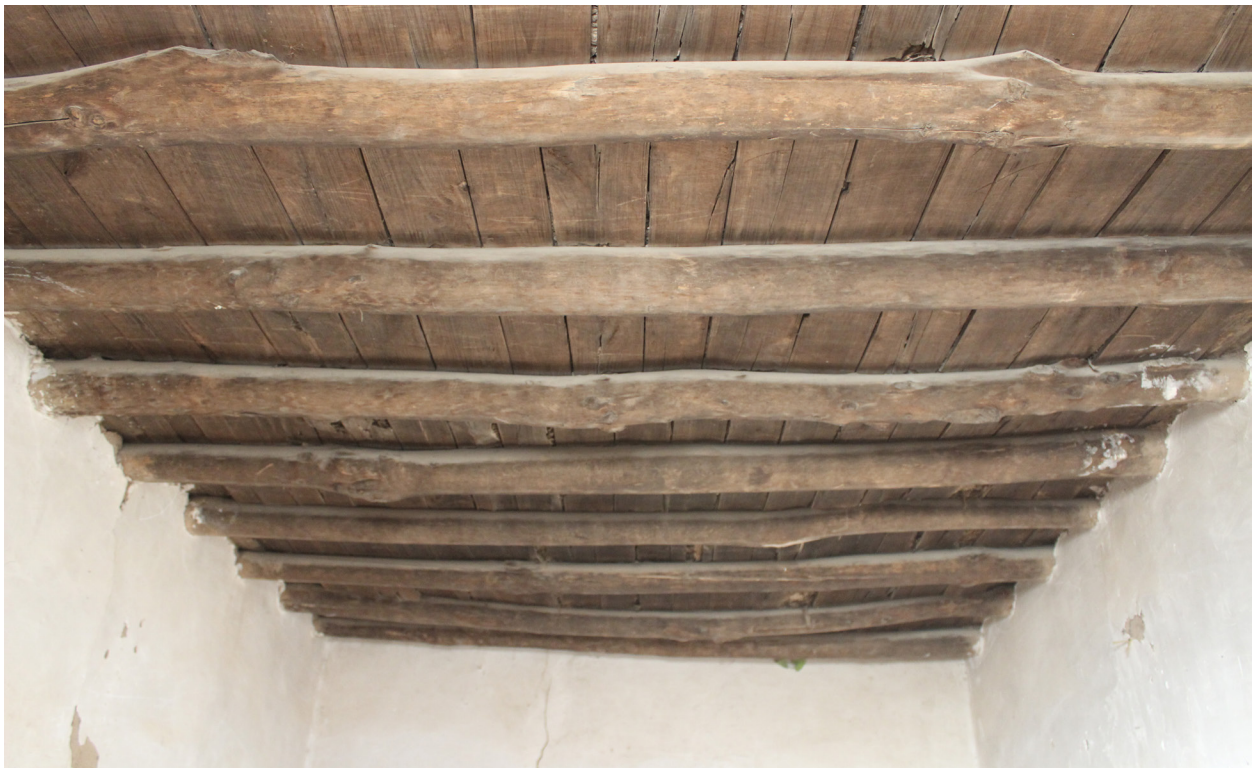
Figure 60 Abandoned house in Jazan
