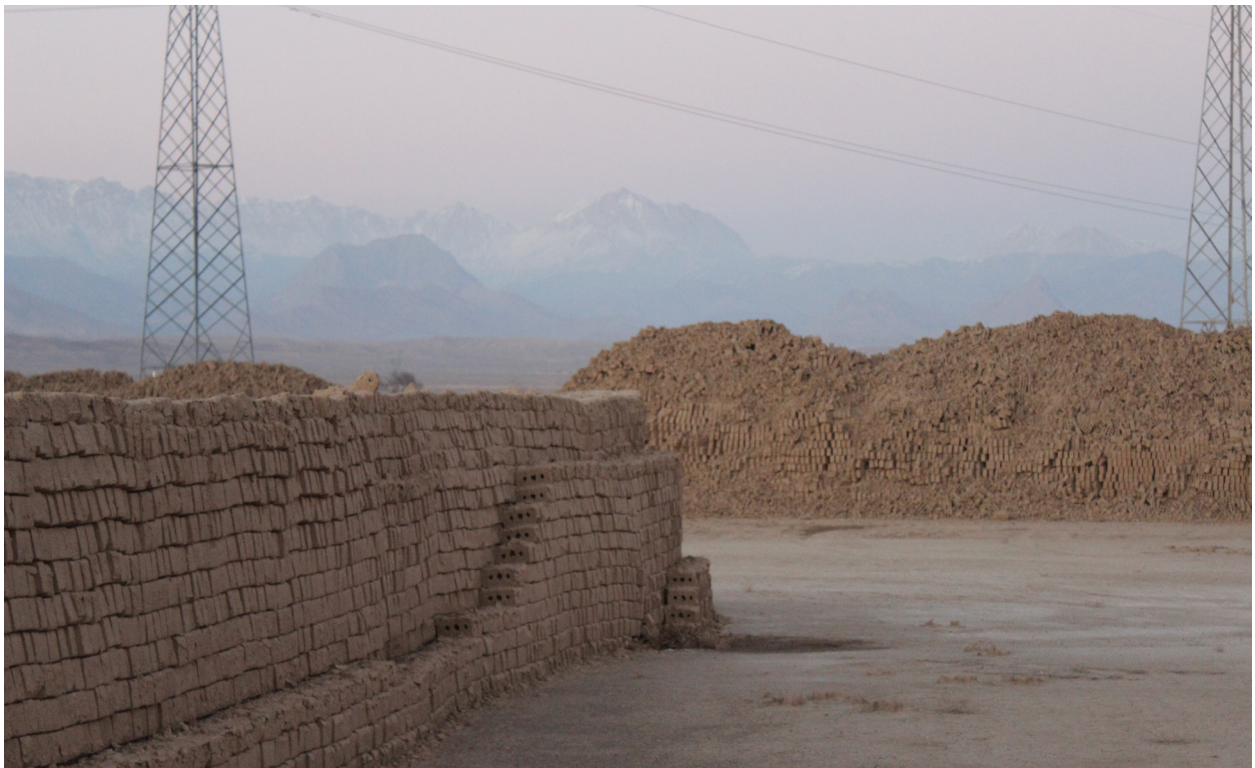
Figure 78 Unfired brick storage around the kiln
