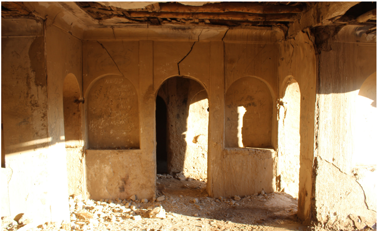
Figure 58 Abandoned house in Jazan
