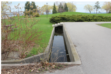
Fig. 133. Photo of water channel, 2019.
