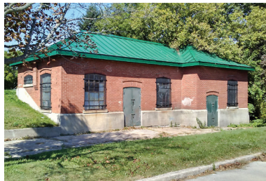
Fig. 130. Photo of water treatment facility, 2018.
