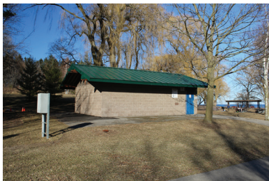
Fig. 98. Photo of washrooms, 2019.
