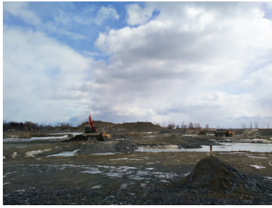
Fig. 193. Soil remediation at 70 Mississauga Road South, 2018.
