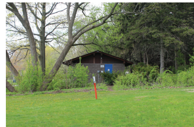
Fig. 82. Photo of washrooms, 2019.
