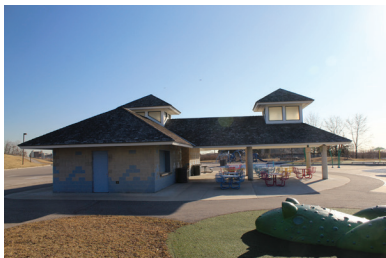
Fig. 112. Photo of washrooms / changerooms, 2019.
