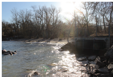
Fig. 95. Photo of channelized creek outlet, 2019.
