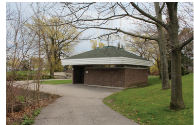
Fig. 131. Photo of washrooms, 2018.
