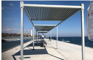
Fig. 48. Photo of pier covered shelter, 2019. (Photo courtesy of Michelle Dalcourt)
