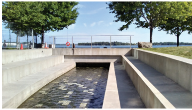
Fig. 66. Photo of concrete water channel carrying clean water to Toronto's Inner Harbour beyond, 2018.
