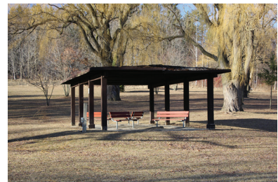
Fig. 100. Photo of covered shelter, 2019.
