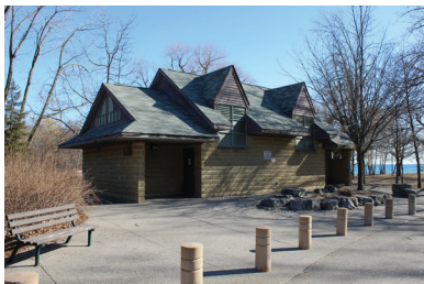
Fig. 84. Photo of washrooms, 2019.
