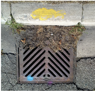
Fig. 70. Photo of a painted yellow fish stencil next to a typical catch basin cover in Mississauga, 2019.
