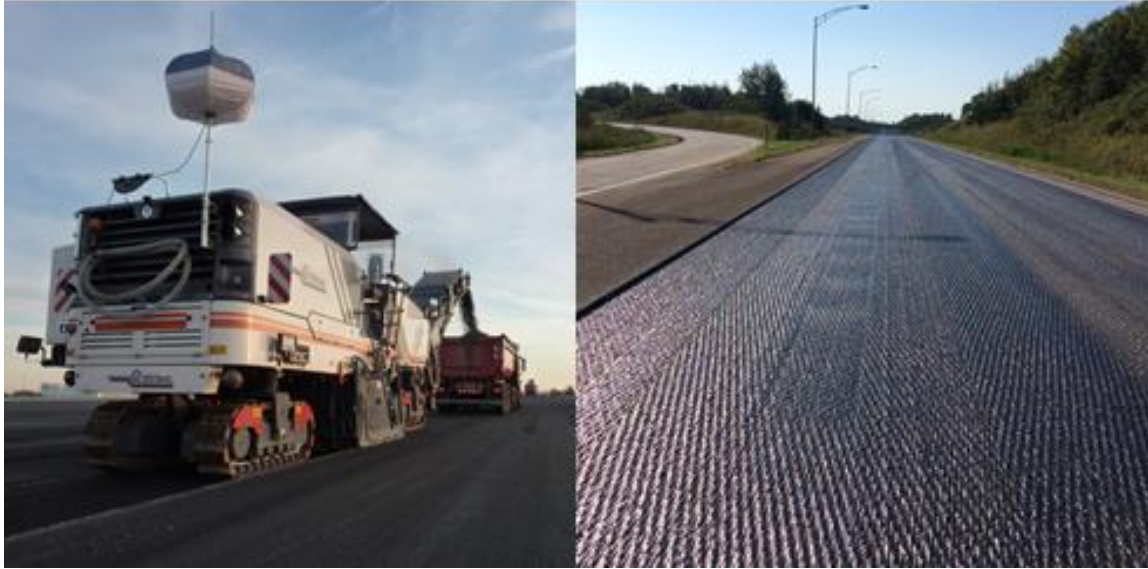
Figure 3.6: Left – Asphalt Milling Machine, Right – Milled Surface (Cleaver 2016)
