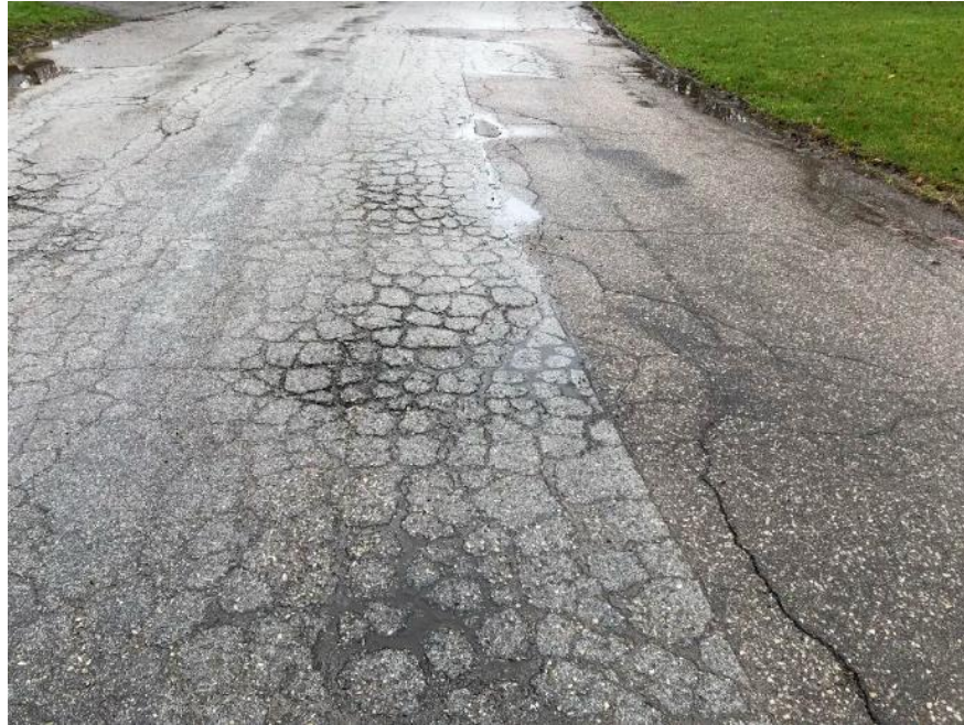
Figure 4.7: Saw-Cut and Repaired Area, Taken May 8 th , 2019
