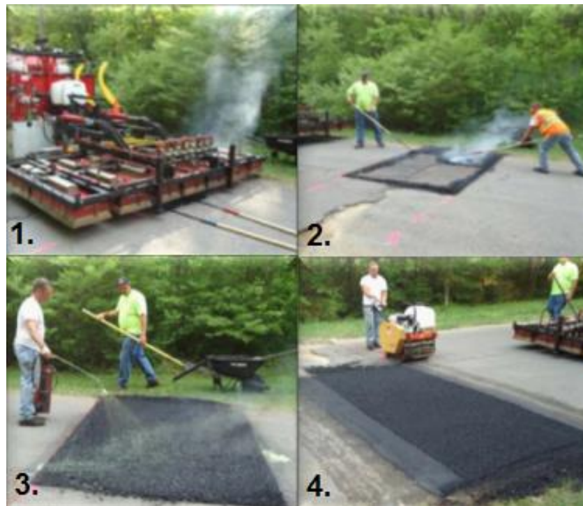
Figure 1.2: 1) Infrared Heating 2) Scarifying 3) Rejuvenators Added 4) Compaction (Kieswetter 2013)
