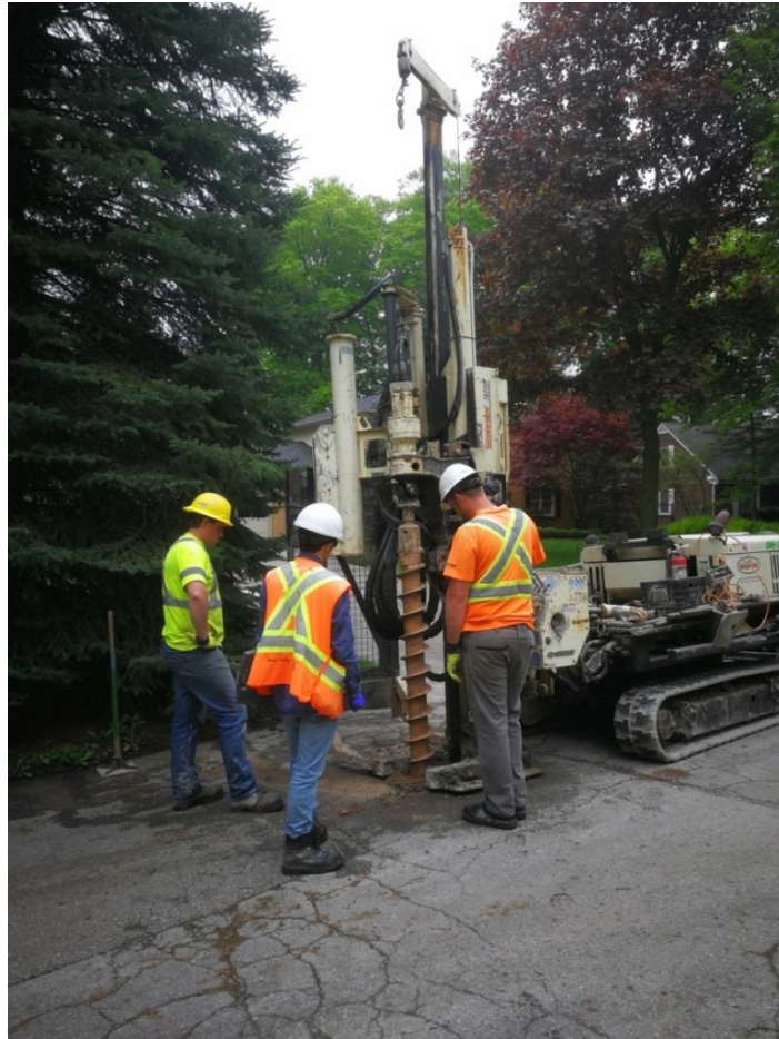
Figure 4.18: Auger Drilling on Sugarbush Drive, Taken May 30 th , 2019
