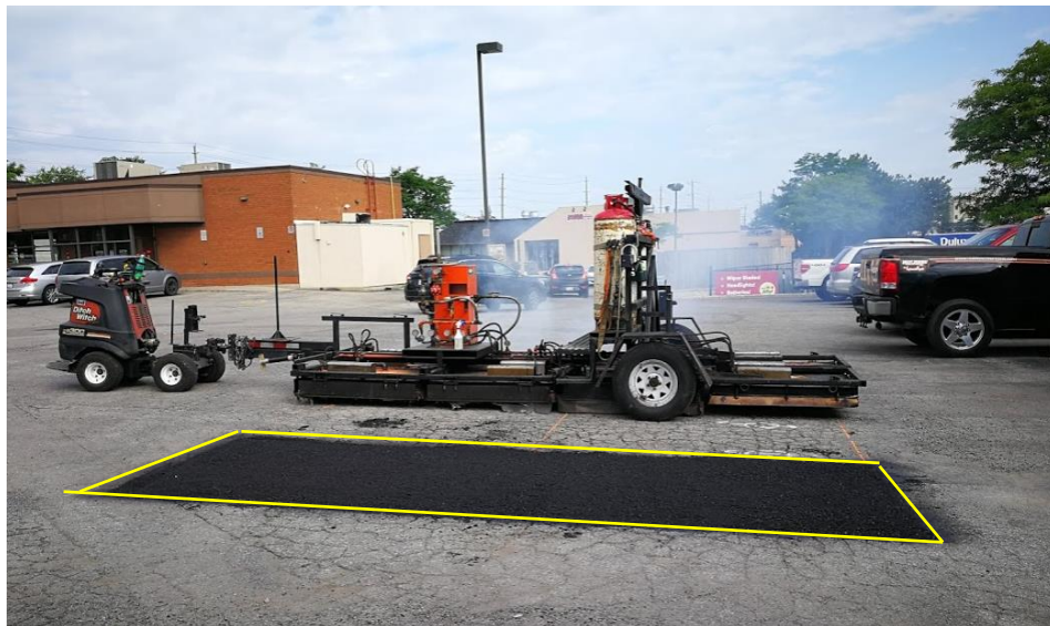
Figure 3.9: Fresh Infrared Heating Patch Repair
