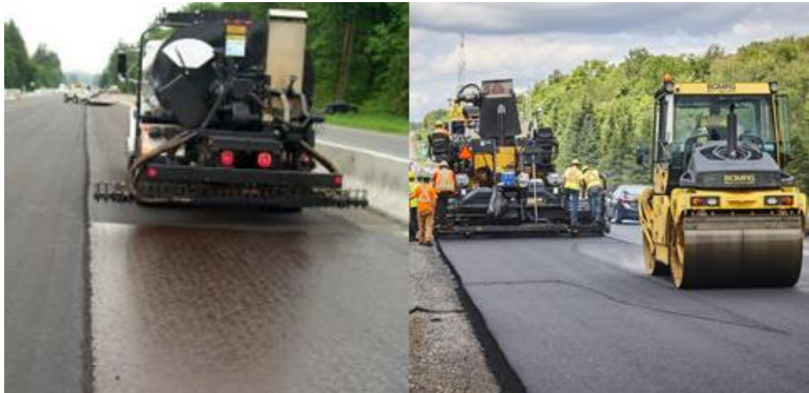
Figure 3.7: Left – Application of Tack Coat (Pavement Interactive 2019b), Right – Paving and Compaction (Fowler Construction 2019)
