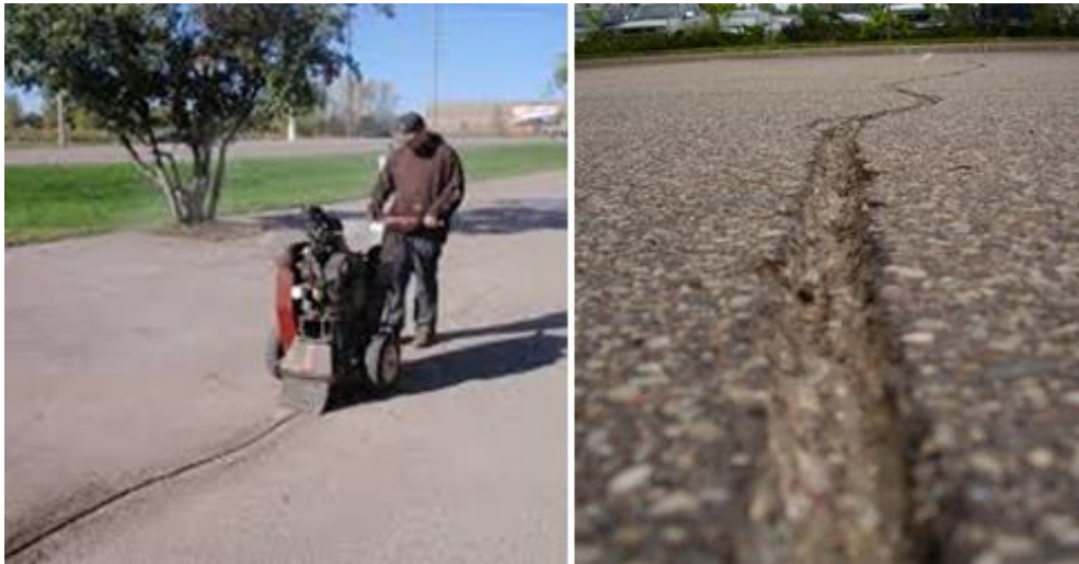
Figure 3.3: Left – Crack Routing Machine in Use, Right – Routed Crack (Brahney 2015)
