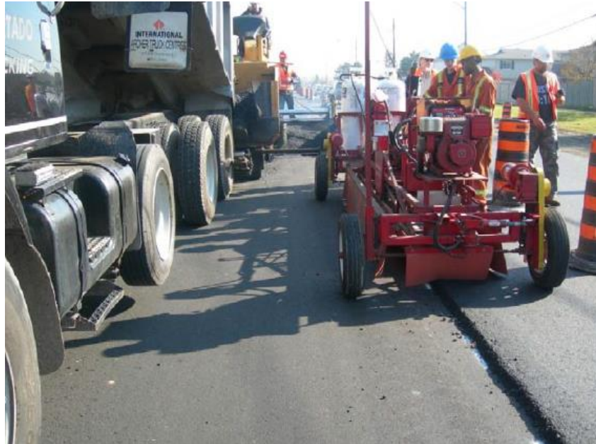
Figure 2.2: Placement of Surface Course Using Infrared Joint Heater on Rymal Road, Hamilton in 2008 (Uzarowski et al. 2009)
