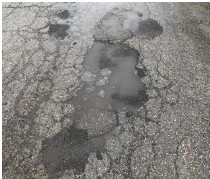
Figure 4.6: Patched Areas of Sugarbush Drive, Taken May 8 th , 2019
