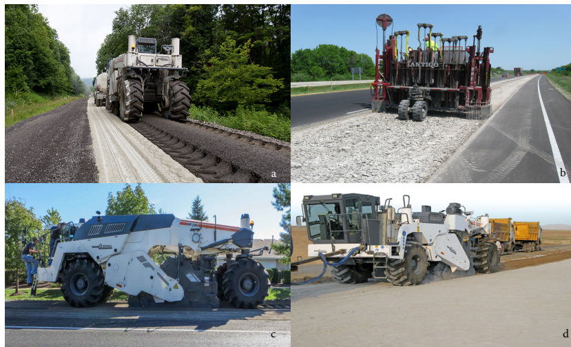
Figure (2.5) Roadway Rehabilitation Activities 3
