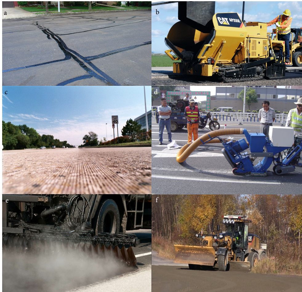
Figure (2.4) Roadway Preservation Activities 2
