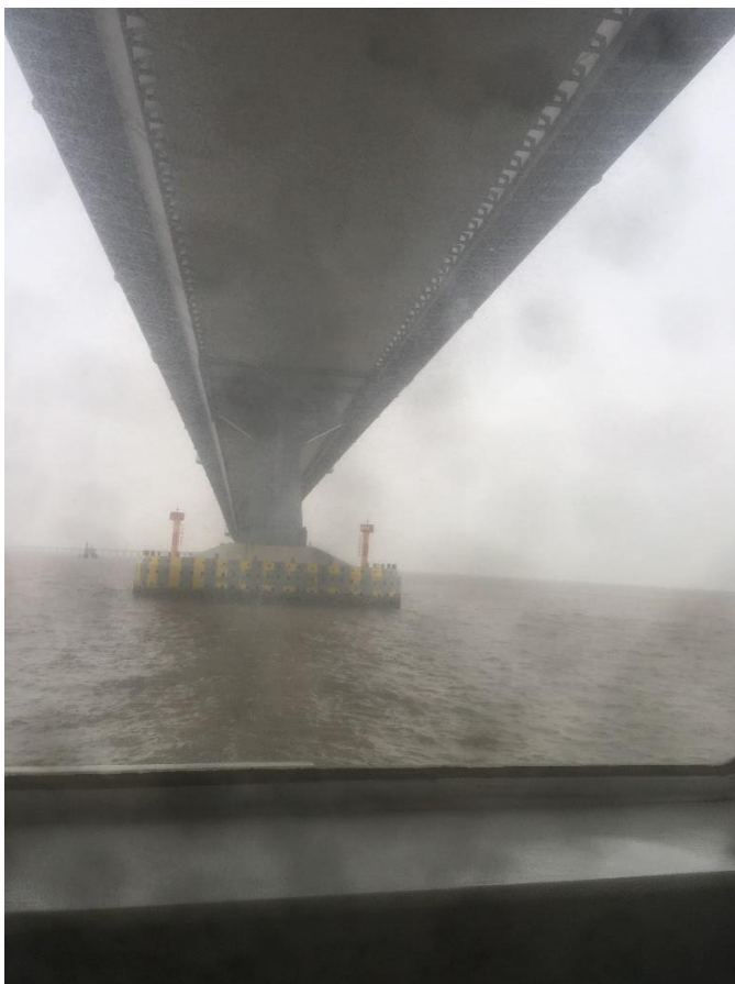
Figure 4.3 Hong Kong-Zhuhai-Macao Bridge; taken directly beneath it in a boat.
