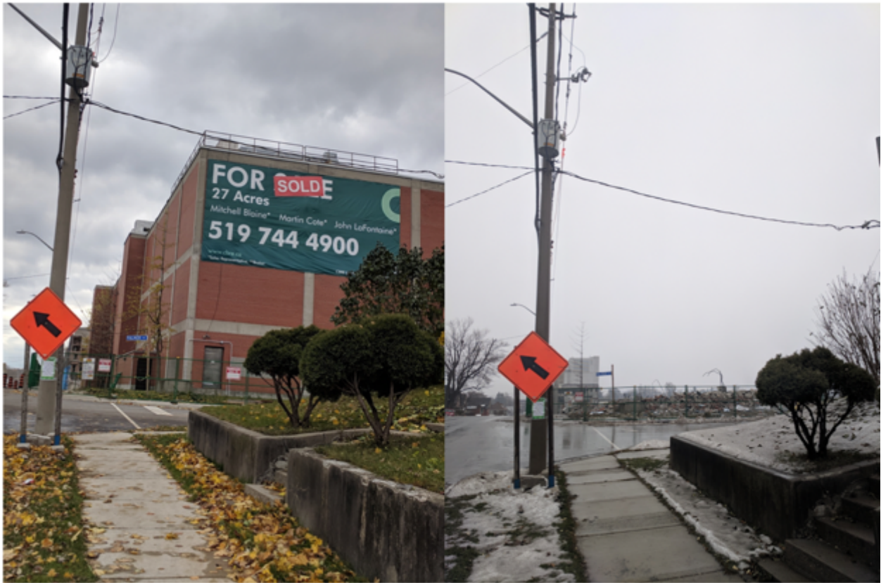
Figure 5-10: Schneiders (2018). Pre-redevelopment and post-demolition.
