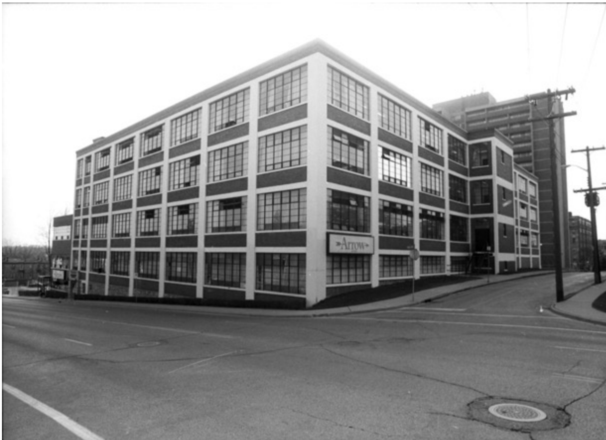
Figure 5-19: Arrow Shirt Factory (1983)
