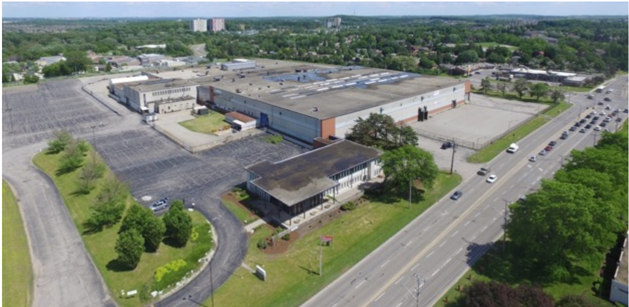
Figure 5-16: Aerial view of former Lear Automotive plant from Manitou Drive (2016)
