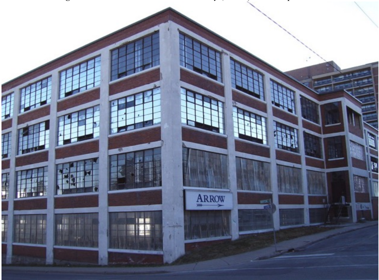
Figure 5-20: Former Arrow Shirt Factory (~2003), Pre-adaptation.
