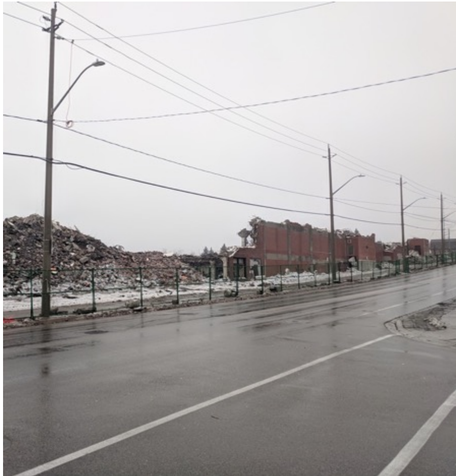
Figure 5-9: Schneiders factory demolition (2018)
