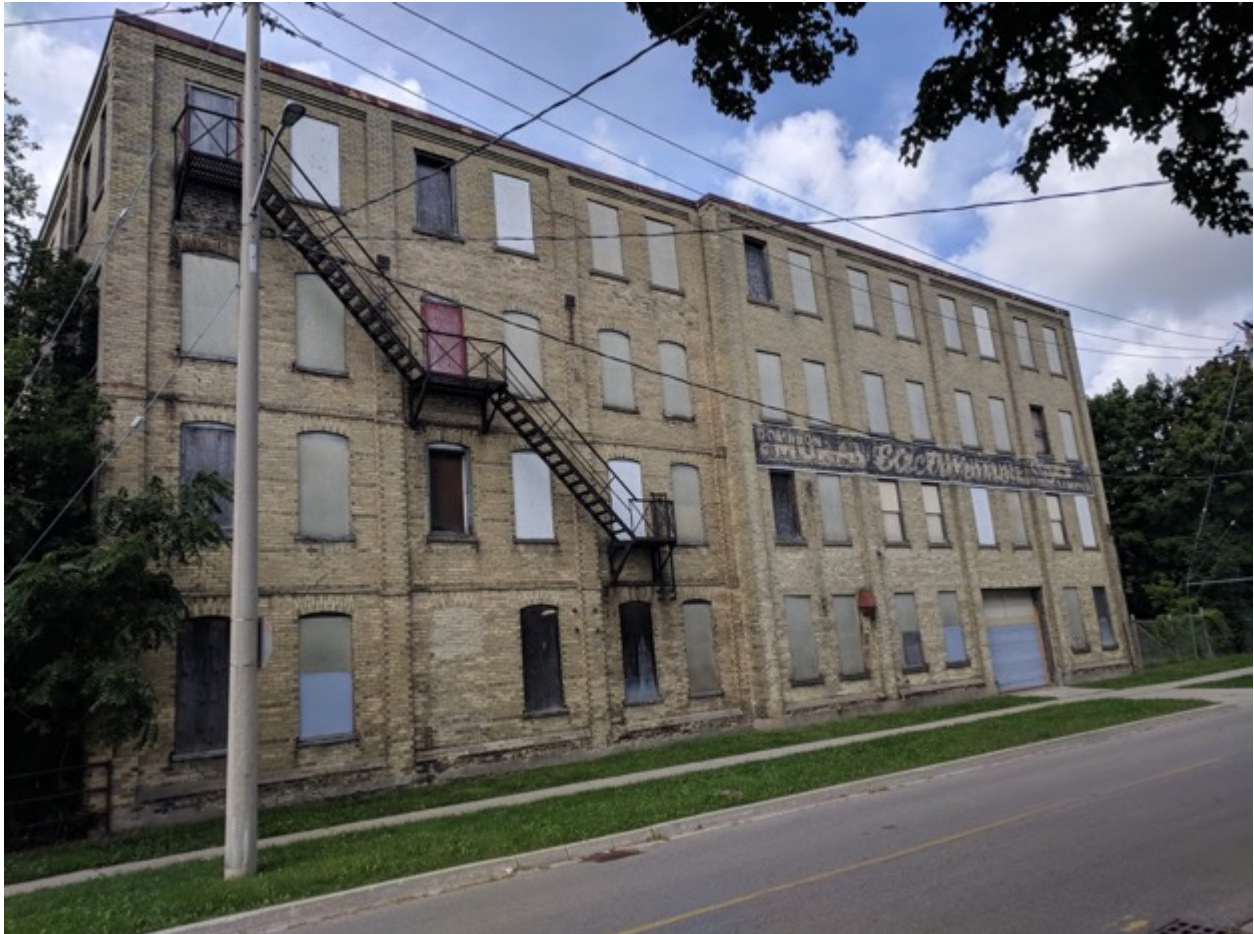
Figure 5-23: Abandoned former Electrohome building (2018)
