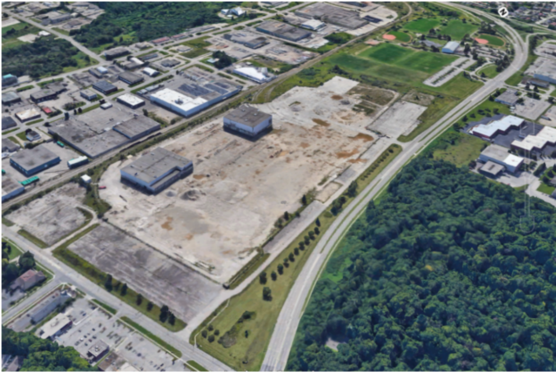
Figure 5-13: Aerial of former Budd Automotive site (2018)
