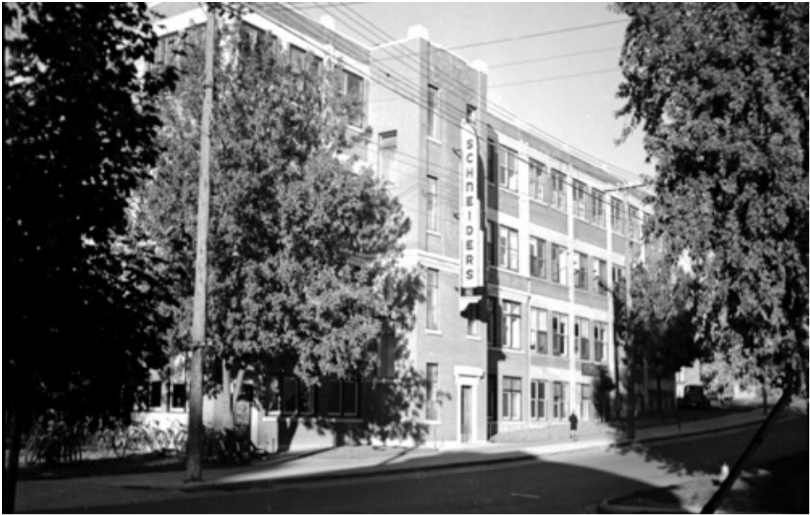
Figure 5-7: Schneiders' former main entrance (n.d.)
