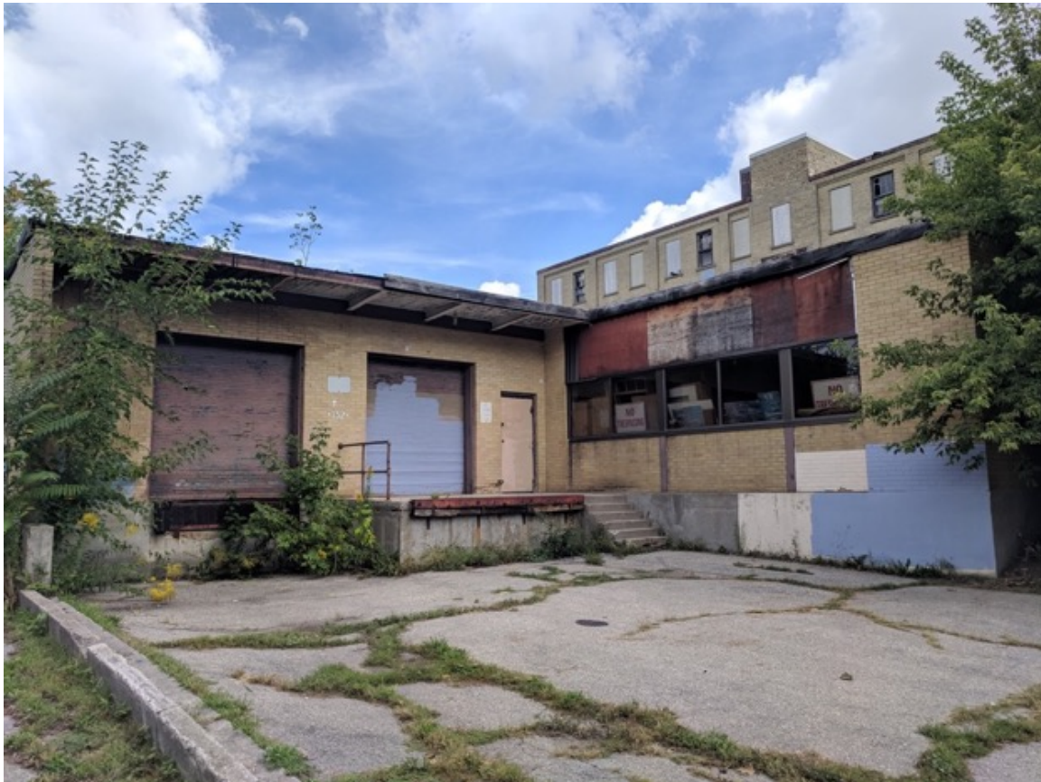
Figure 5-24: Abandoned former Electrohome building (2018)
