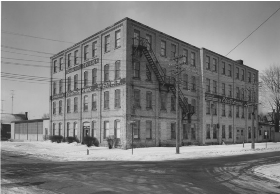
Figure 5-22: Electrohome plant (n.d.)
