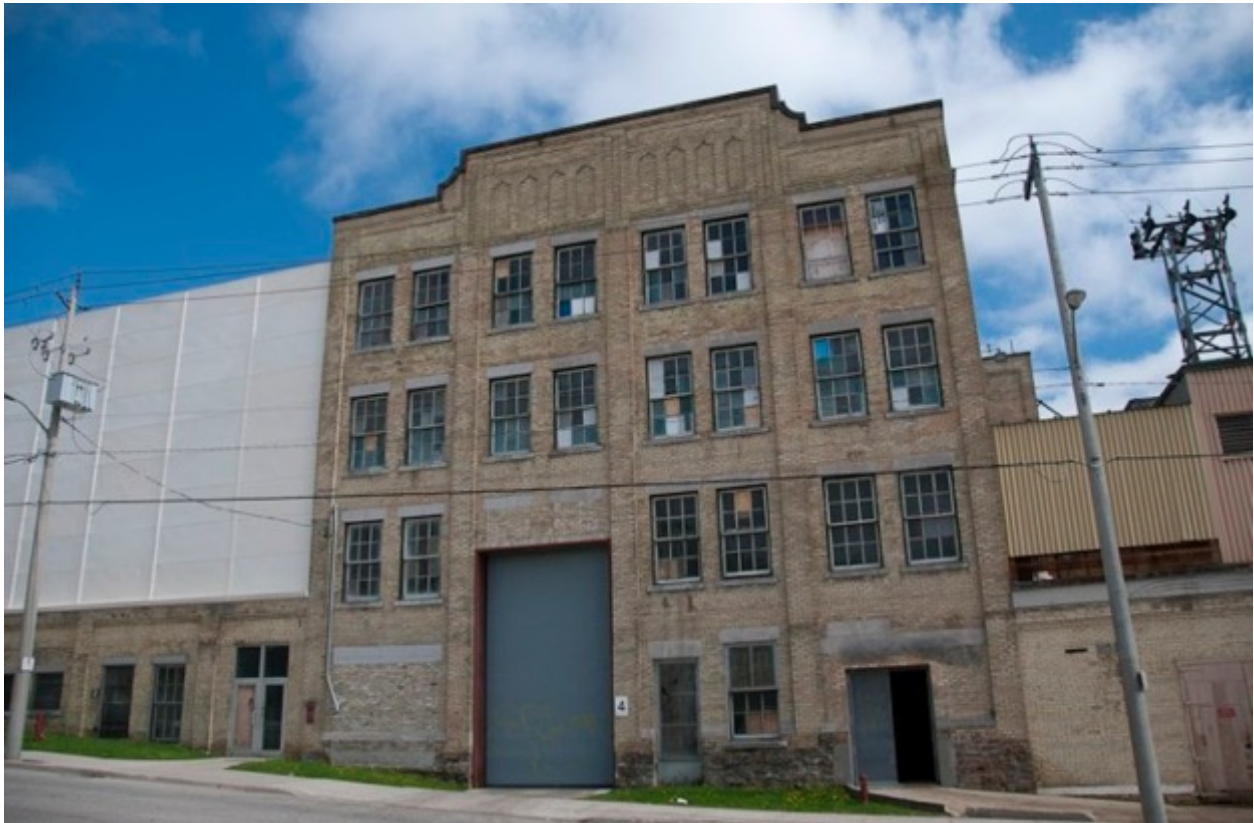
Figure 5-14: Former Dominion Rubber site, pre-adaptation (2012)
