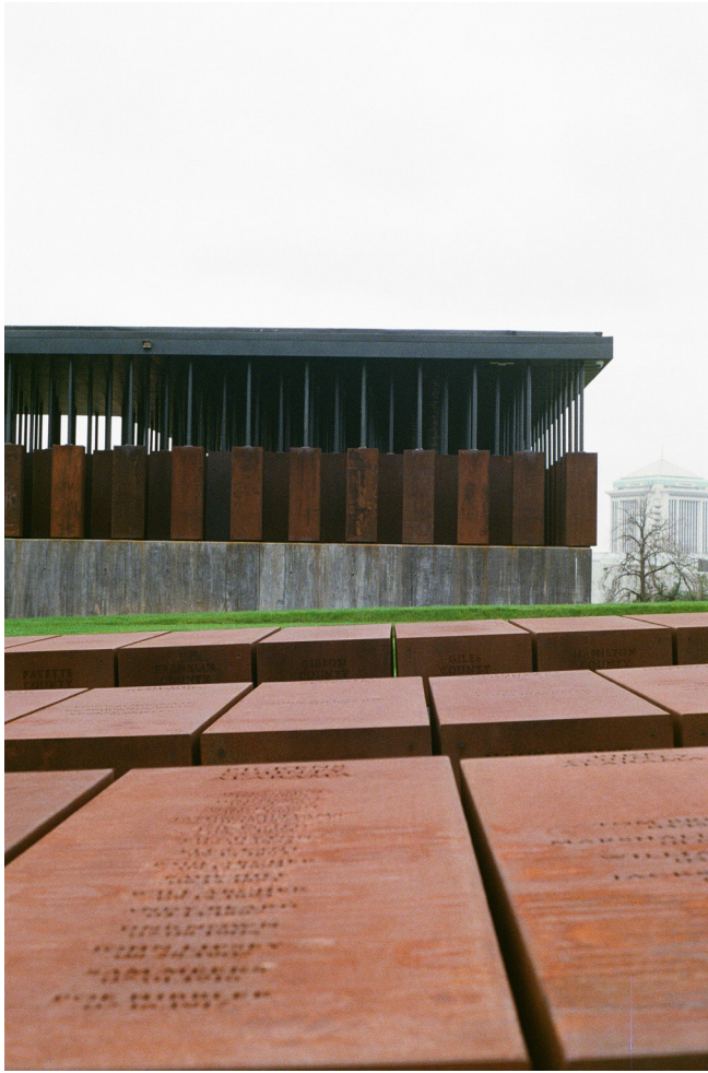
Figure 3.4.12: South side from memorial park.
