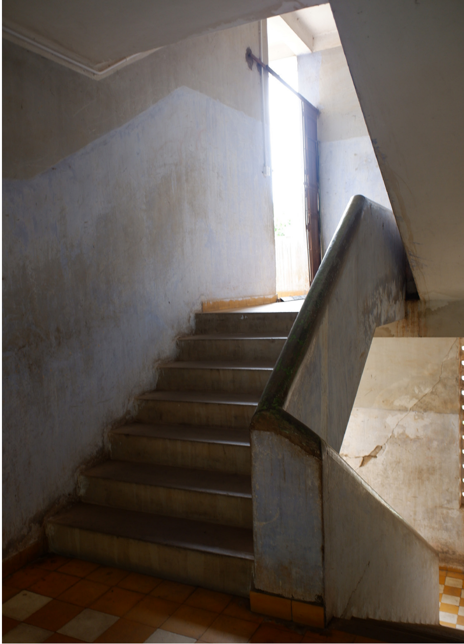
Figure 3.2.17: Staircase in Block A.
