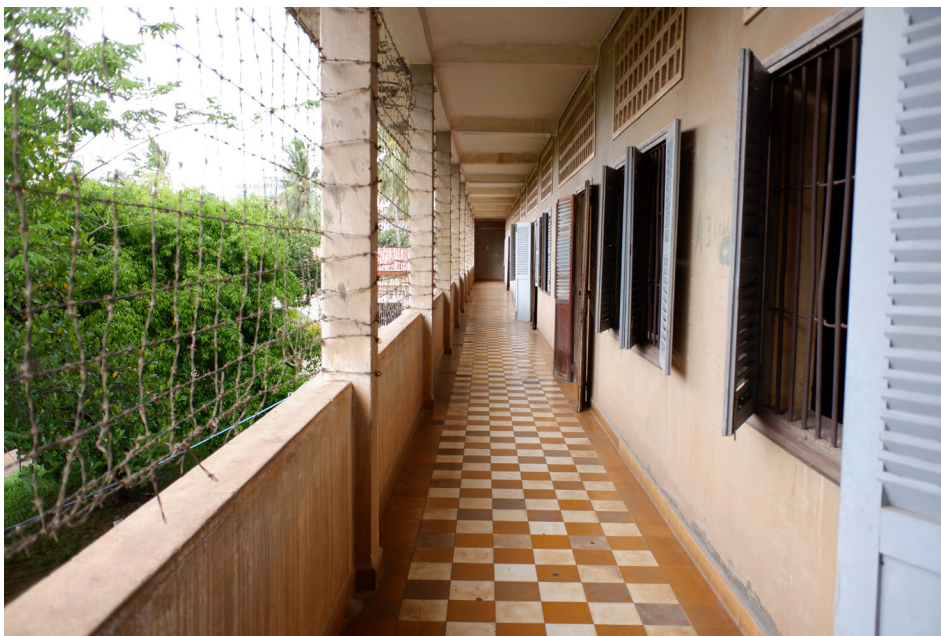
Figure 3.2.3: Corridor in Block C.
