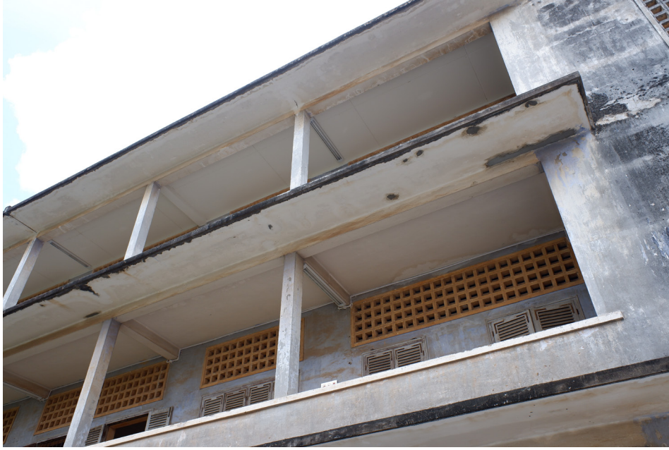
Figure 3.2.12: Block A from below.
