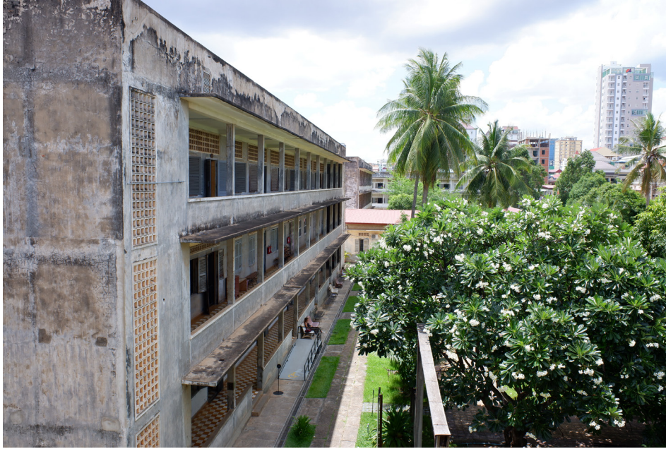
Figure 3.2.5: Block B from Block A.
