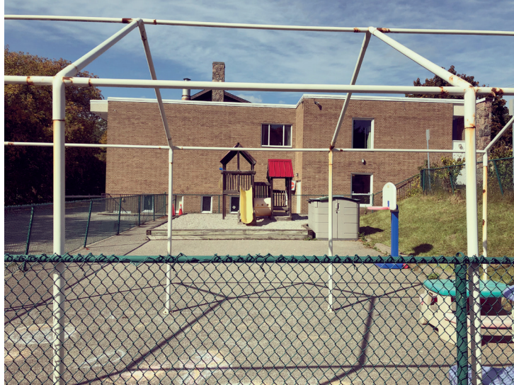
Figure 68. Current playground at the childcare facility, East view
