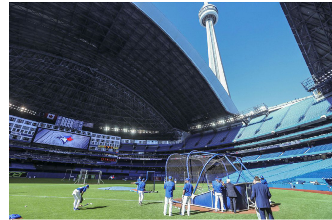
Figure 1.1.20 The Roof of the Rogers Center in Toronto opens and closes to provide outdoor or indoor experiences depending on the exterior conditions.
