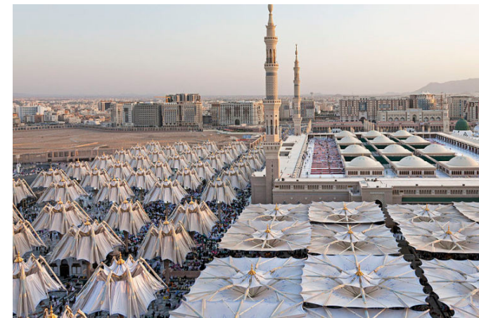
Figure 1.1.19 The Umbrellas in Medina opens and closes to open up the space as well as offer environmental protection depending on the weather and time of day.
