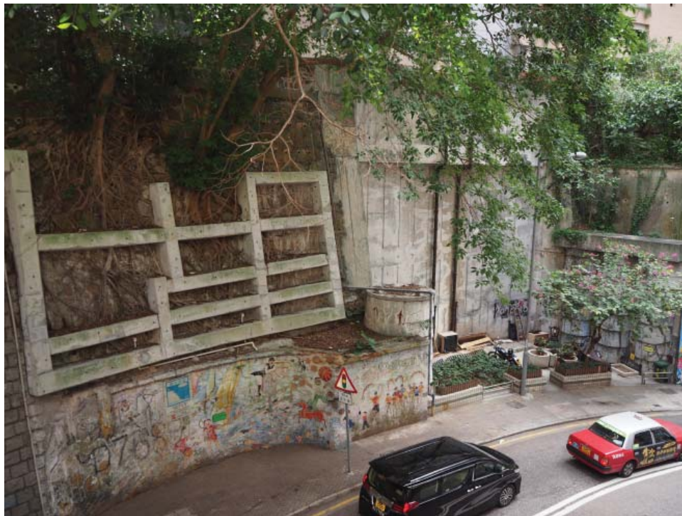
Figure 4.28 Mid-Levels retaining walls and environments
