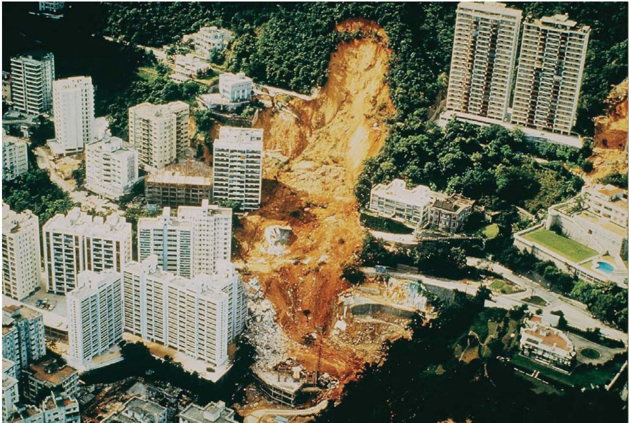
Figure 4.2 Aerial Photograph of the 1972 landslide at Kotewell Court, Mid-Levels, Hong Kong
