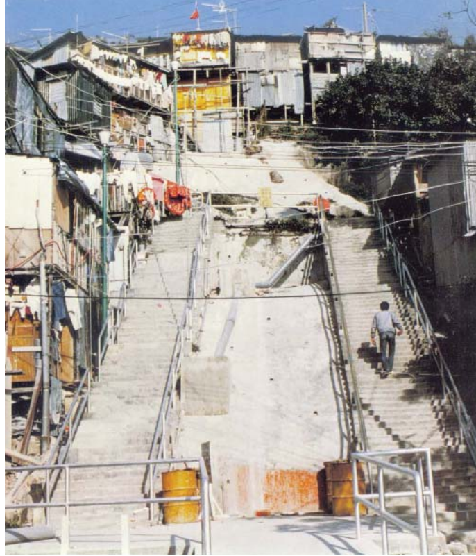
Figure 4.22 Fire break in a squatter community
