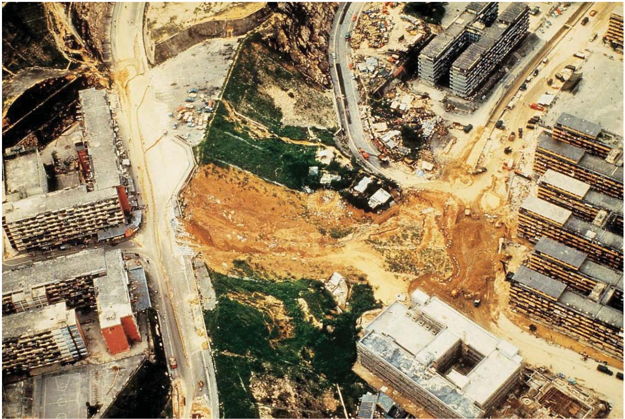
Figure 4.1 Aerial Photograph of the 1972 landslide at Sau Mau Ping, Kwun Tong, Hong Kong
