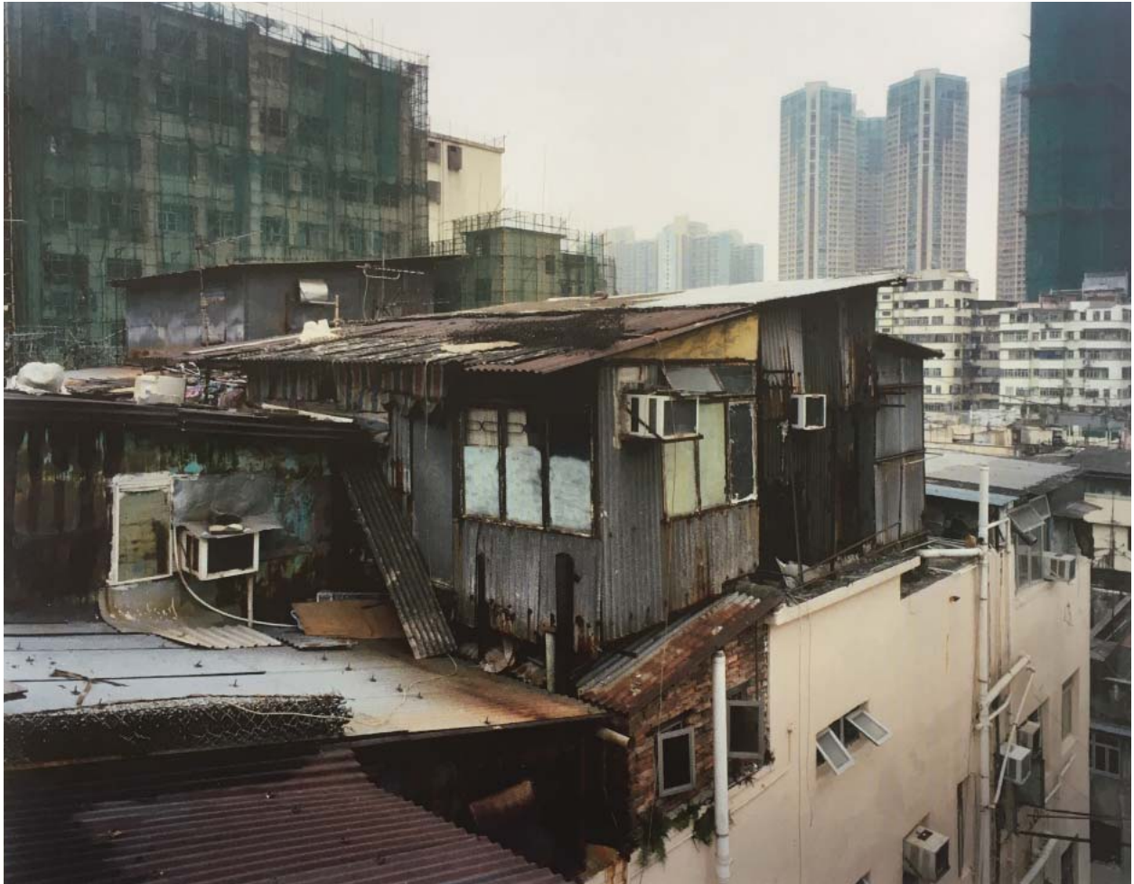
Figure 2.12 Informal Rooftop Settlement
