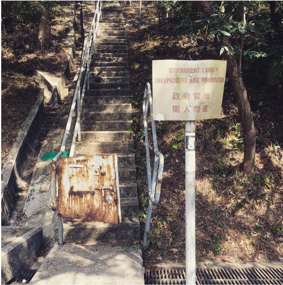
Figure 4.4 Gate and sign prohibiting the use of slopes
