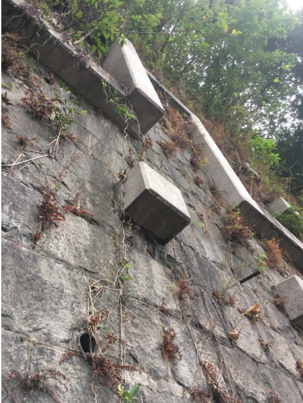
Figure 4.8 Soil nail in a retaining wall
