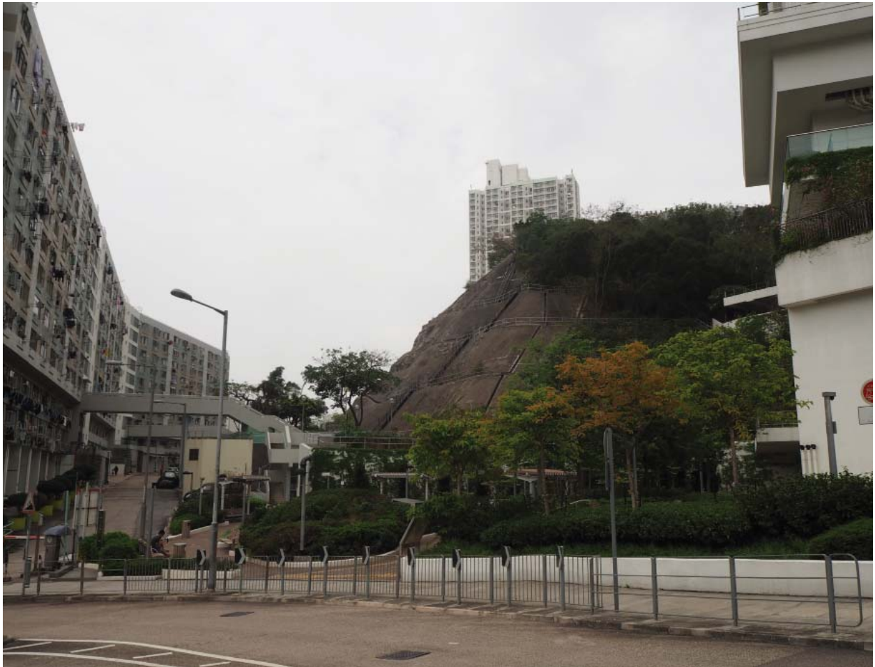
Figure 5.9 The Mei Tung Estate Slope
