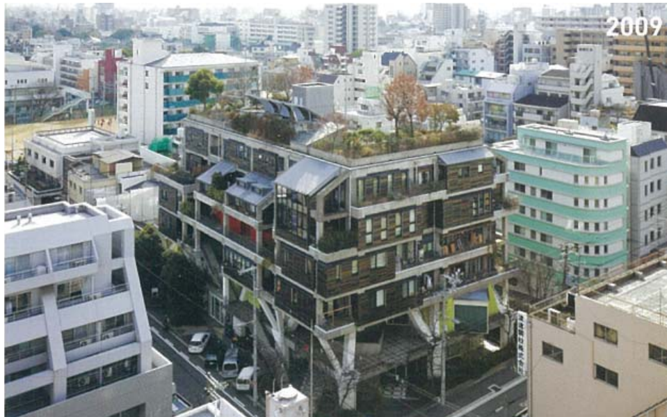
Figure 3.10 Next21 Exterior View
