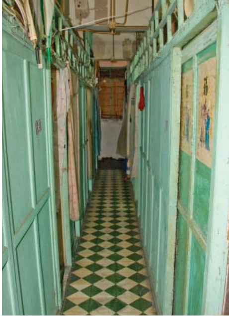
Figure 2.7 Corridor in a sub-divided unit
