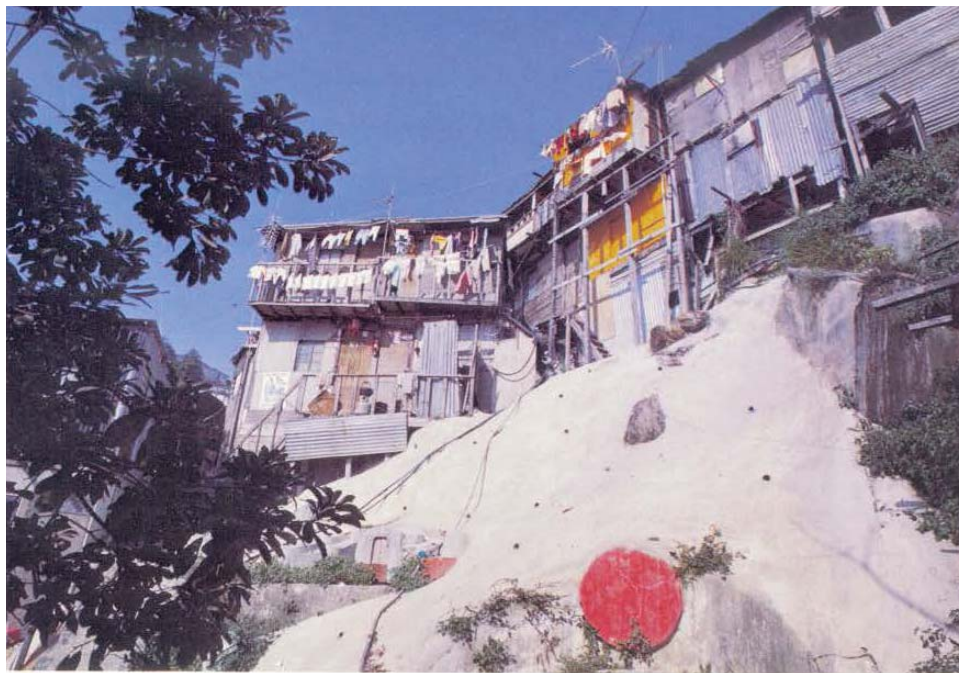
Figure 4.23 Slope surface improvements in a squatter community
