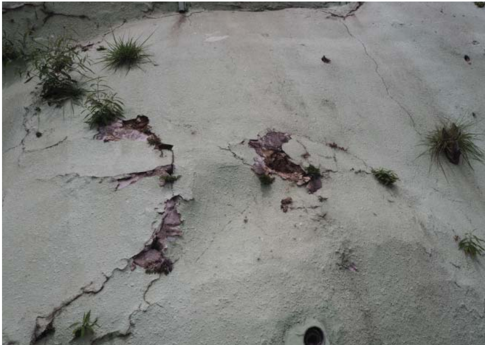
Figure 4.14 Cracking chunam
