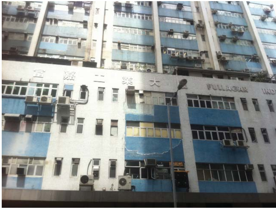
Figure 3.15 Typical Industrial Building Facade
