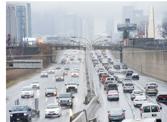
Fig. 1. View looking east along Gardiner Expy. from Lake Shore Blvd. West bridge near Dunn Ave, near peak hour commute
