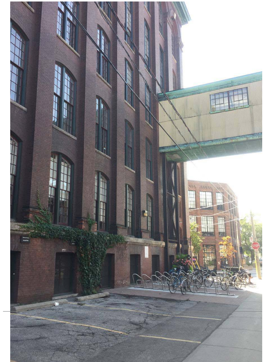
Fig. 24. The Carpet Factory, at grade architectural condition, during non-working hours
