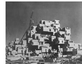
Fig. 5. Habitat by Moshe Safdie for Expo 67, under construction in Montreal, QC
