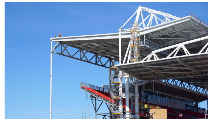
Fig. 37. BMO Field phase two canopy and seating construction, ongoing
