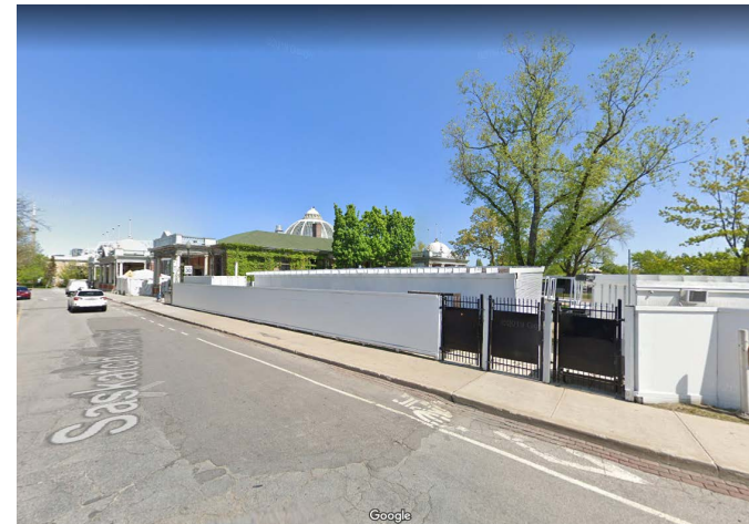
Fig. 35. Public-to-private barrier surrounding the Horticulture Building
