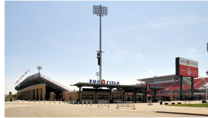
Fig. 36. BMO Field complete after phase one construction
