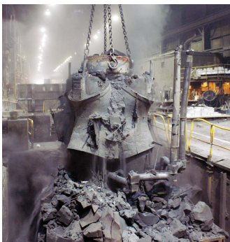
Fig. 73. Queen Richmond Centre West, node casting by CAST CONNEX
