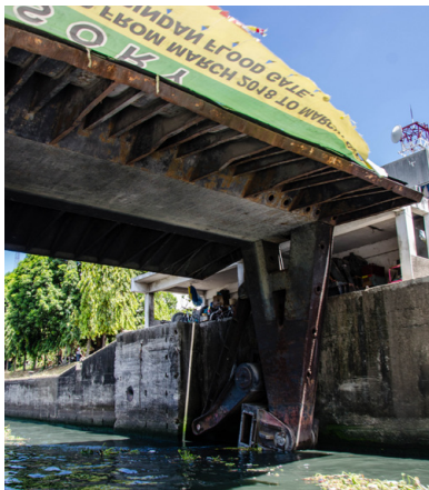
fig. 3.20 Under an open lock of the Napindan Hydraulic Control Structure. Makati.
