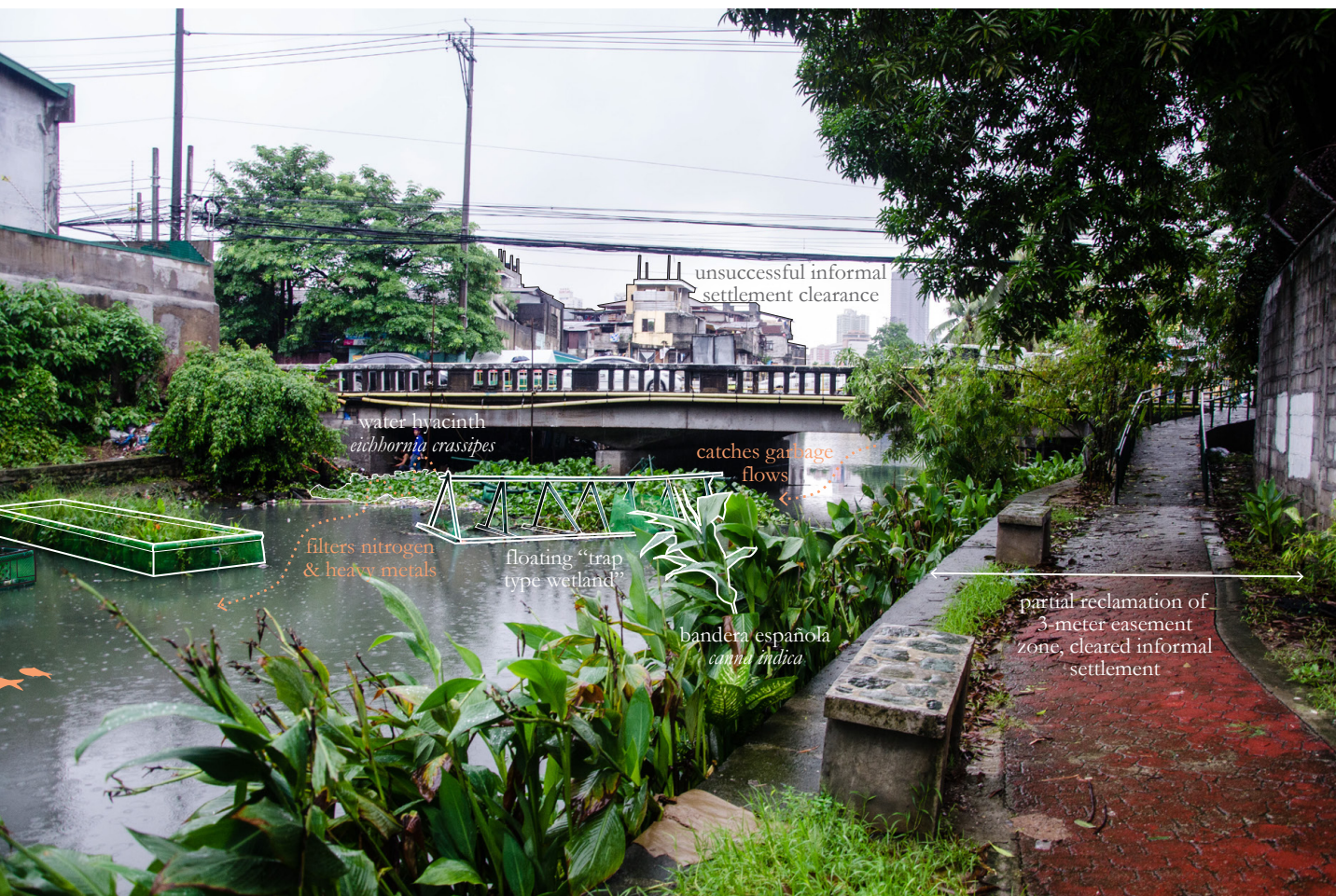
fig. 3.45 Techniques used in the Estero de San Miguel revitalization. Manila. (below)
