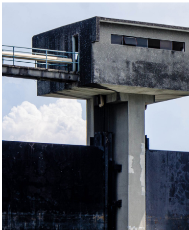
fig. 3.19 Tower on the main Napindan Hydraulic Control Structure. Makati.
