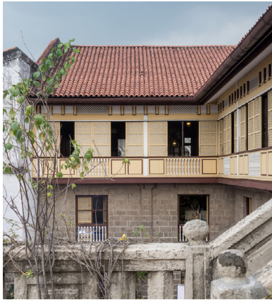
fig. 1.21 Restored bahay na bato of stone and nipa (reproduction) in the Casa Manila complex. Intramuros, Manila.
