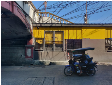
fig. 3.26 Jones North, a smaller pumping station. Manila.
