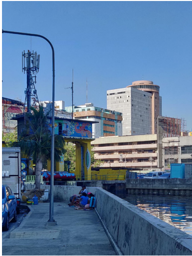
fig. 3.28 Escolta Pumping Station. Manila.
