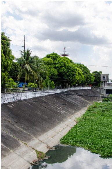
fig. 3.10 Manggahan Floodway's structural wall. Pasig.
