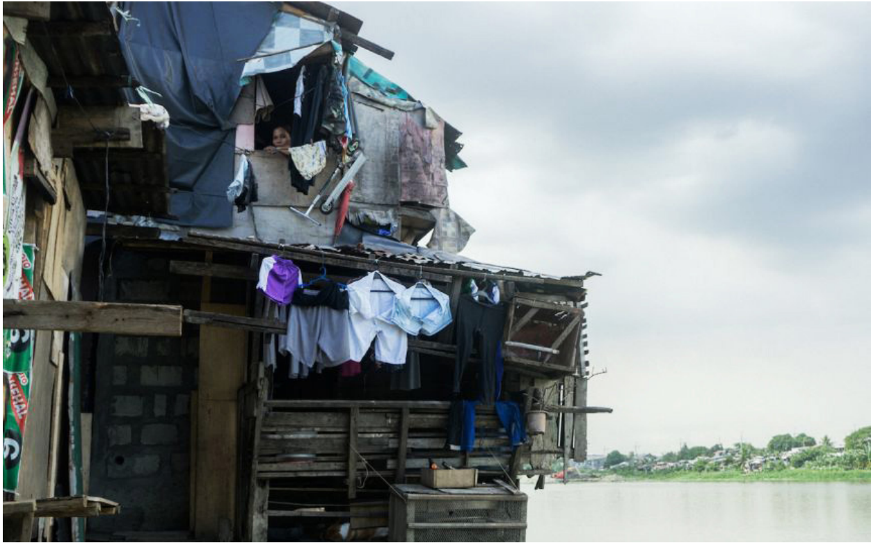
fig. 3.48 Informal housing overhanging the Manggahan Floodway. Pasig.
