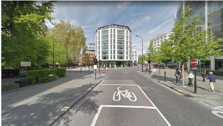
Fig. 5.28 Google maps screen shot of the existing road condition of the West end Cheapside: a predominantly pedestrian & cyclist street with very little vehicular access
