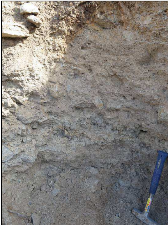
Figure A.15 Sand with granule- to boulder-sized clasts at the Highmont South excavation pit.
