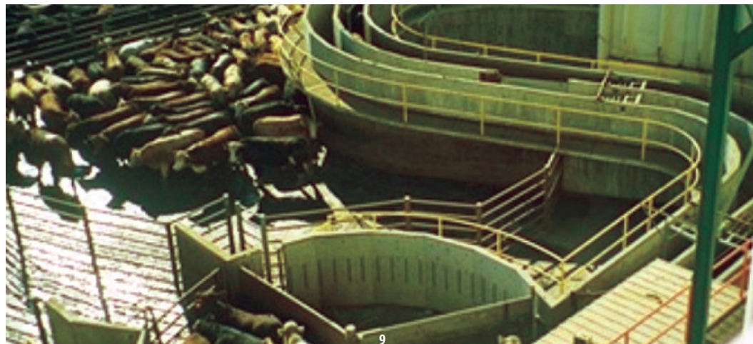
Fig 2.13 Serpentine Ramp, leading from cattle holding pen.
