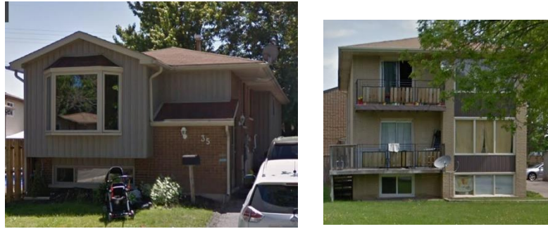
Figure C.1: Photo examples of the building typology classes: Foundation with reinforced concrete and foundation without reinforced concrete.
