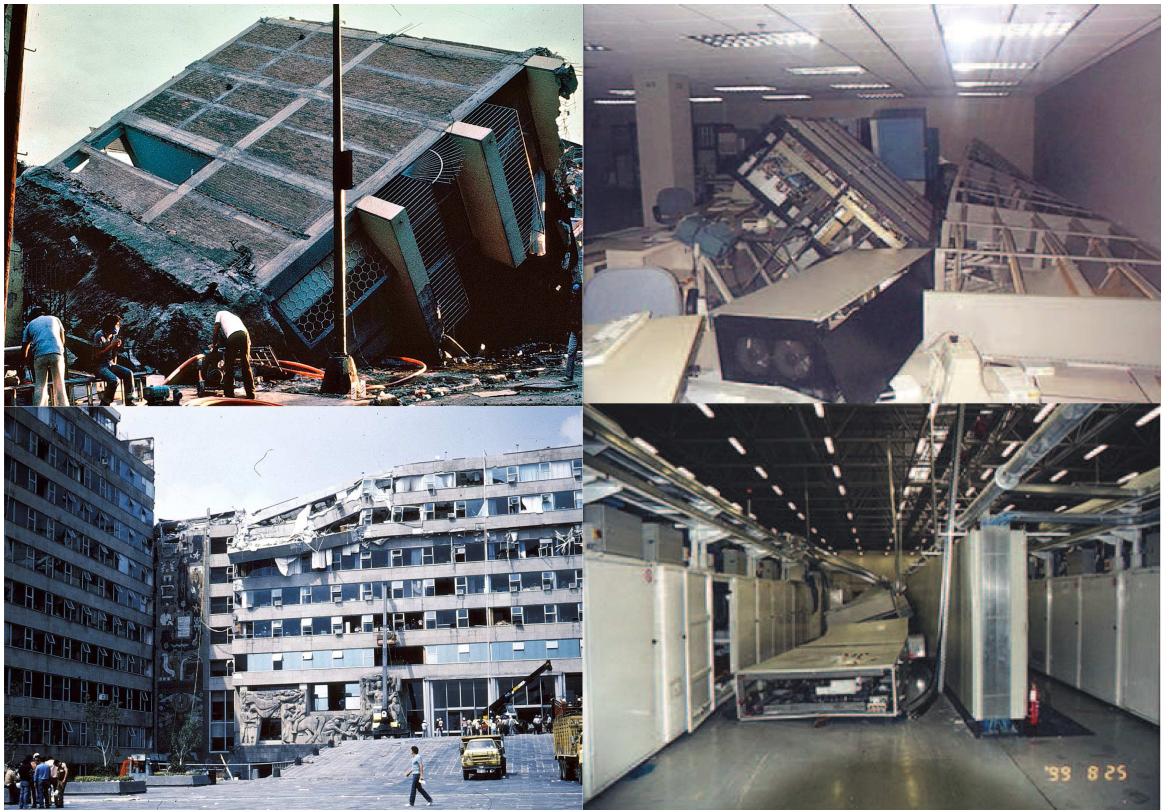
Figure 1.1 Damaged primary structures and secondary system
