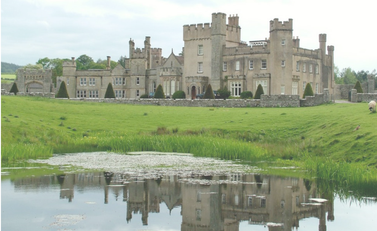
Fig 89. Stanage park, near knighton, powys. The house served, plus some structural prop additions, as handyman hall in the 1985 bbc series of blott on the landscape. © copyright Peter Evans
