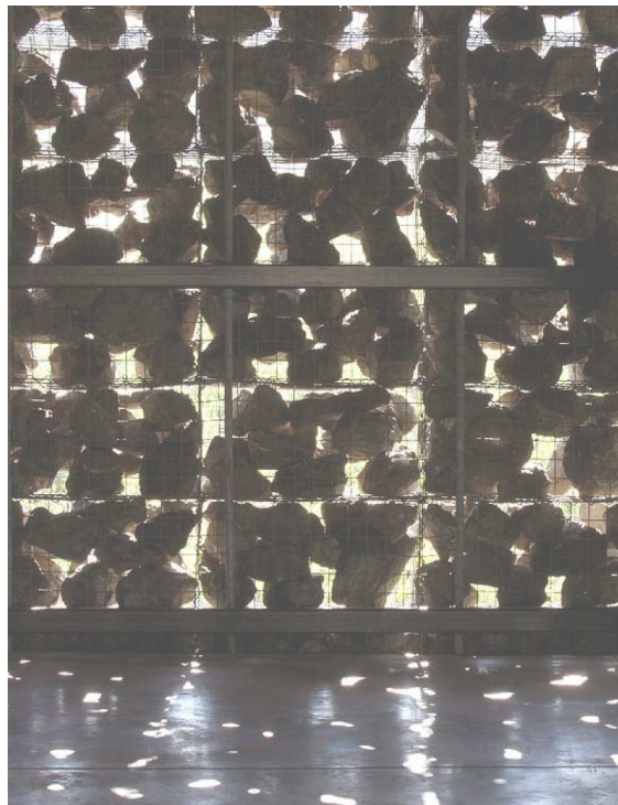
Fig 55. Illustration of Gabion Material – View from Inside the Dominus Winery
