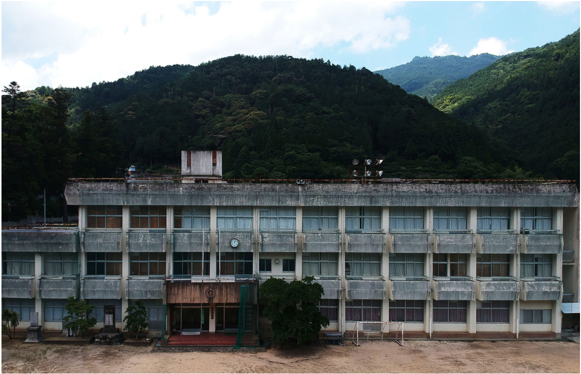
Figure 1.10: A vacant school in Kamiyama, Tokushima Prefecture. The school is built with a typical concrete structure.
