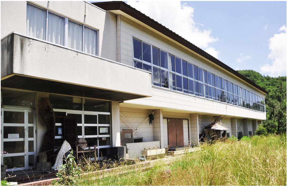
Figure 4.7: The school in its existing condition
