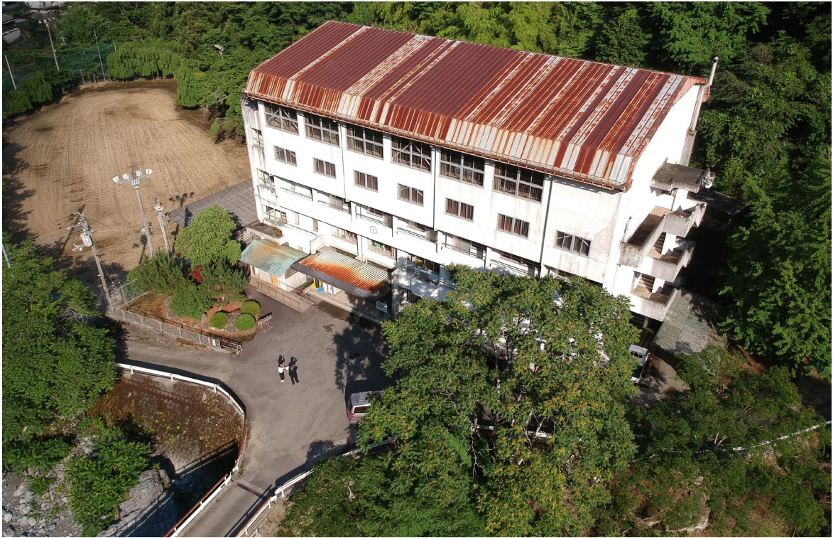
Figure 4.33: Aerial perspective of the selected haiko for Kamiyama. In this building the gymnasium space is stacked on top of three levels of classrooms.
