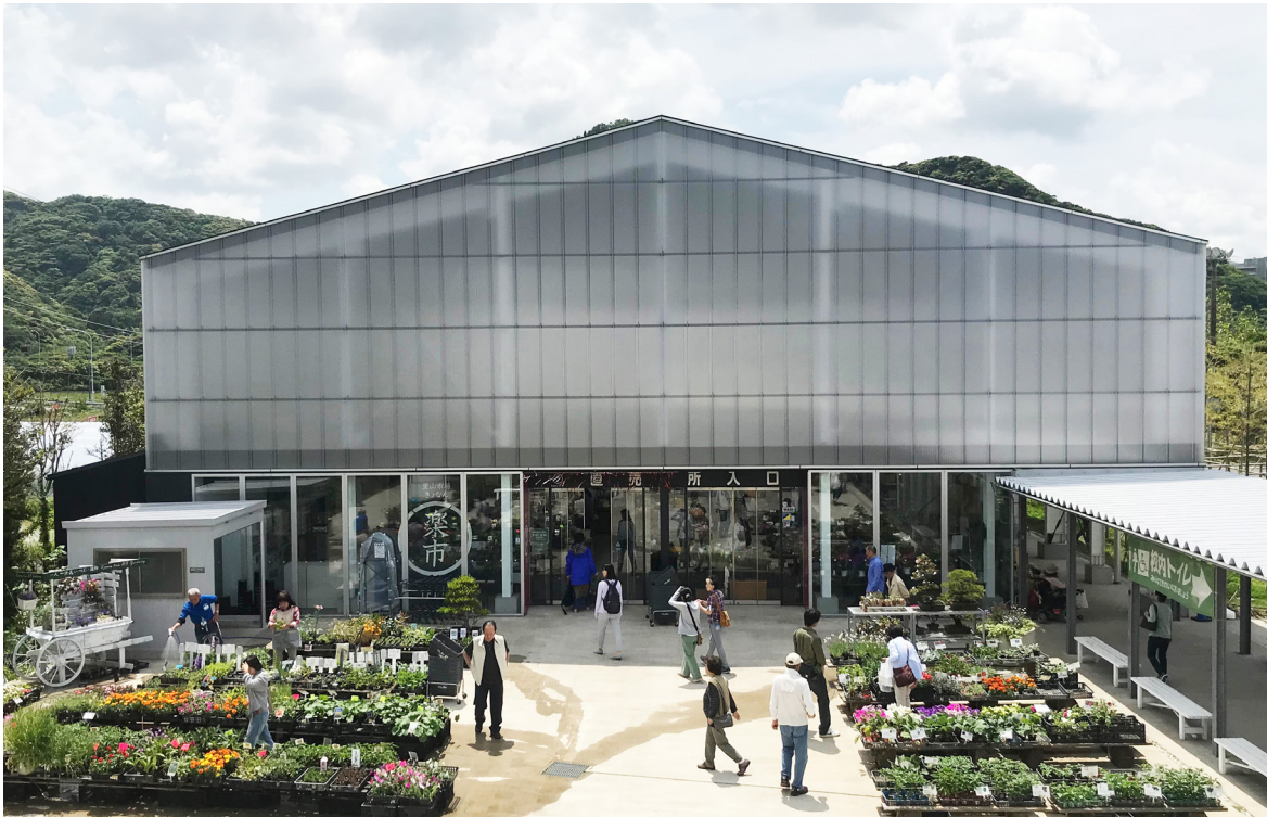
Figure 2.5: The farmer's market at the Hota Road Station. The original gymnasium building of the school has been re-clad in polycarbonate panels.
