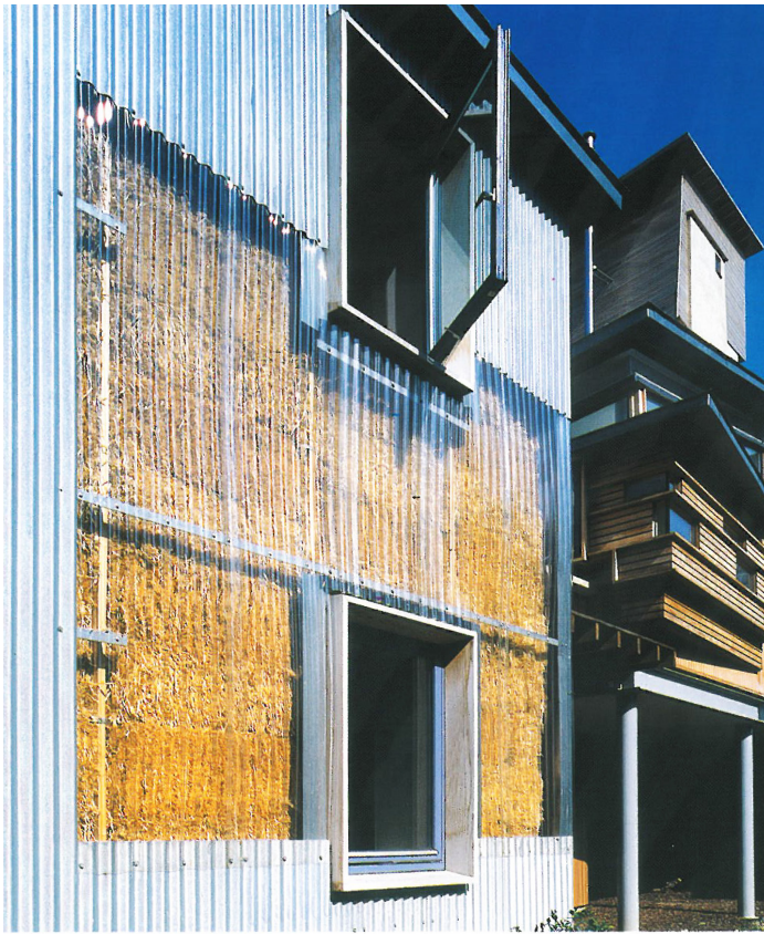
Figure 2.5 Straw Bale House by Sarrah Wigglesworth Architects, 2001. Strawbale Wall Enclosed in Polycarbonate Facade.
