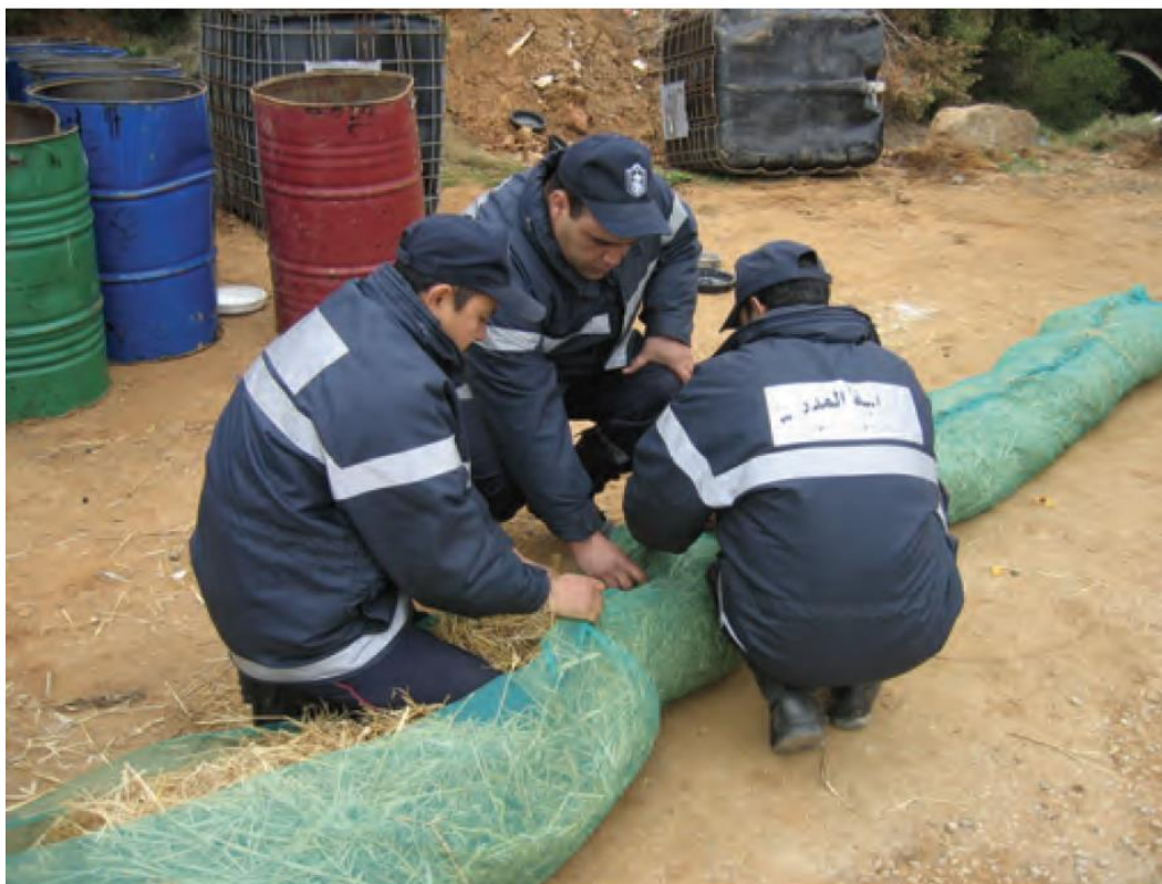
Figure 2.4 Sorbent booms constructed from straw [12].
