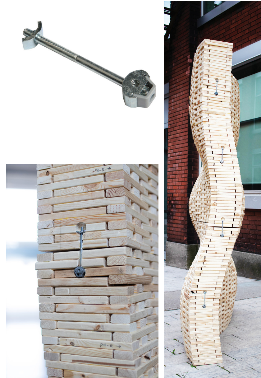
Figure 60. Assembly strategy of fabricated pieces: (top left) Zipbolt that is used as connector; (bottom left) Zipbolt used as connector of two fabricated pieces; (right) final assembled prototype.
