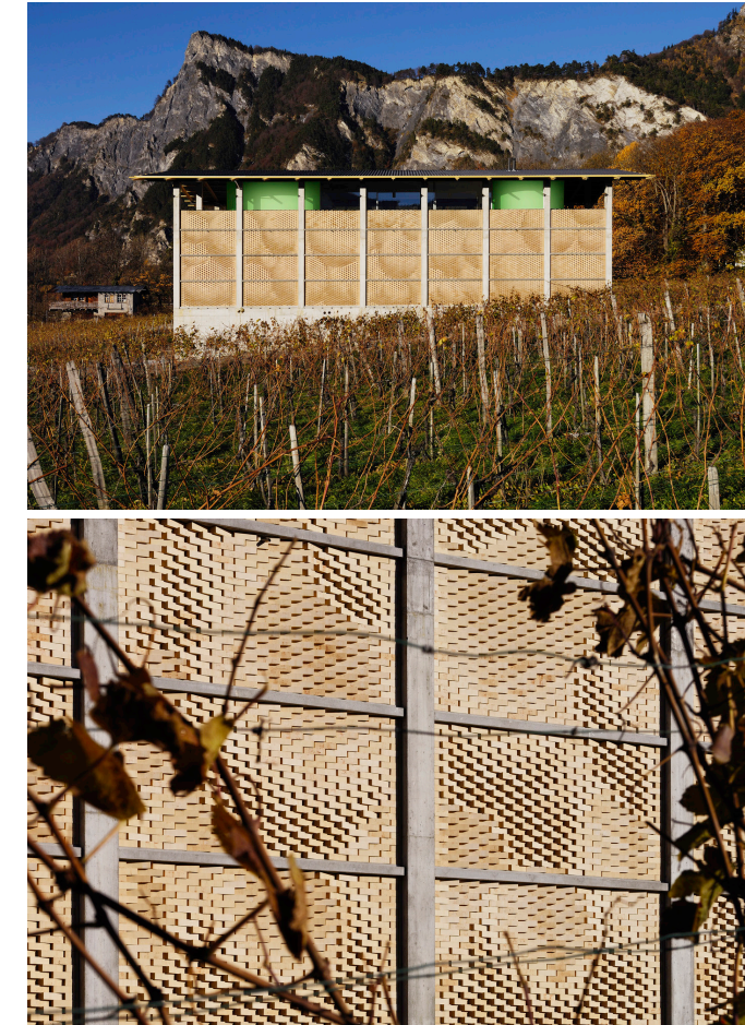
Figure 9. Gantenbein Vineyard Façade, Switzerland, 2006.
