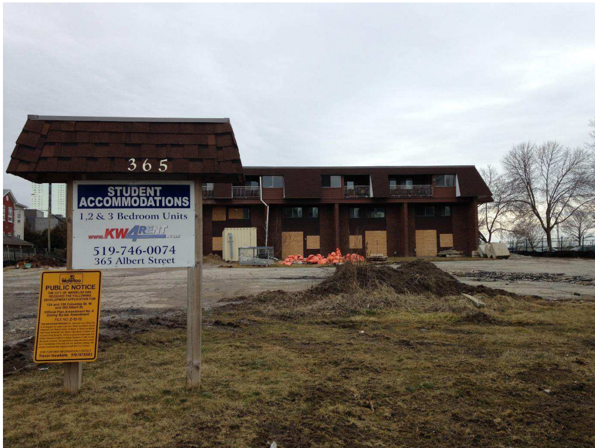
Figure 1.1: Apartment building slated for redevelopment as The Hub, Albert St., February, 2016.
