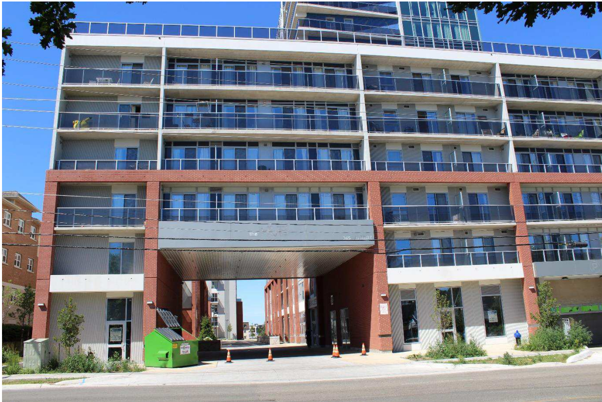
Figure 1.3: The Hub nears completion, July 2018.
