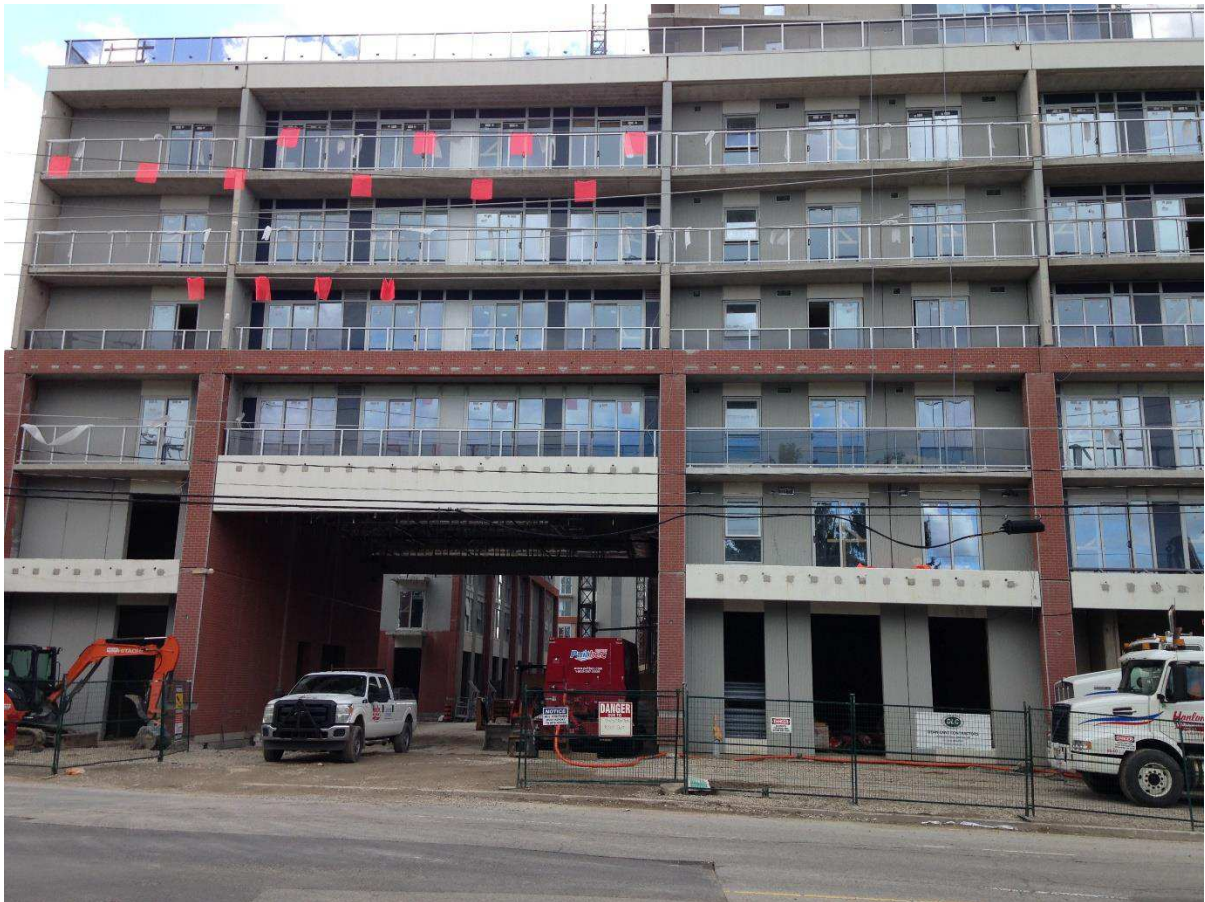
Figure 1.2: The Hub under construction in May, 2017.
