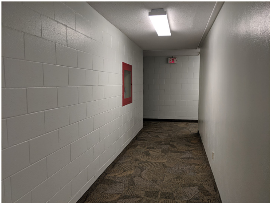
[Fig.32] View of typical corridor at Eby Hall
