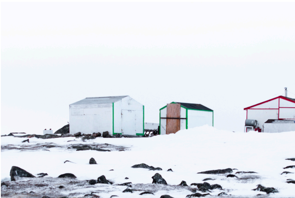
Fig.2.12 Repair shed from the north (top); repair shed and swamp seen together from the northwest (below)
