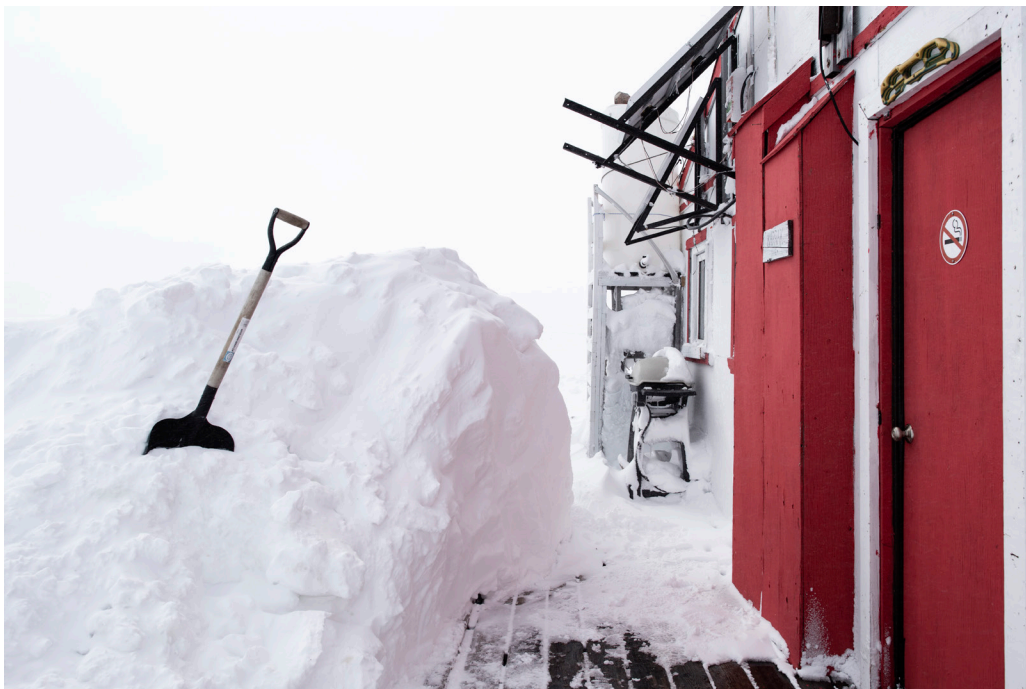
Fig.2.6 Main cabin east facade showing toolshed (top) and looking west down the south facade (below)
