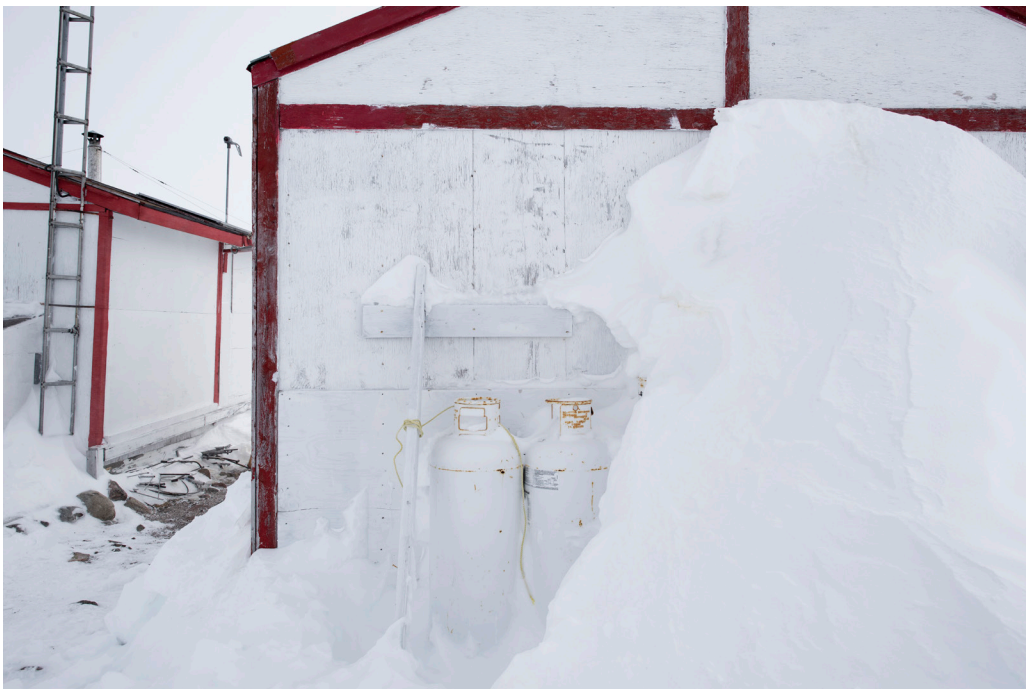
Fig.2.8 Food cabin south (top) and north (below) facades
