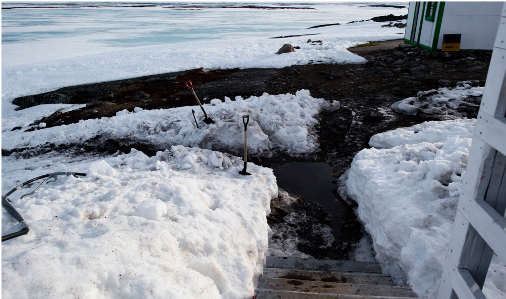
Fig.4.6 Draining water from around the cabins to the lake
