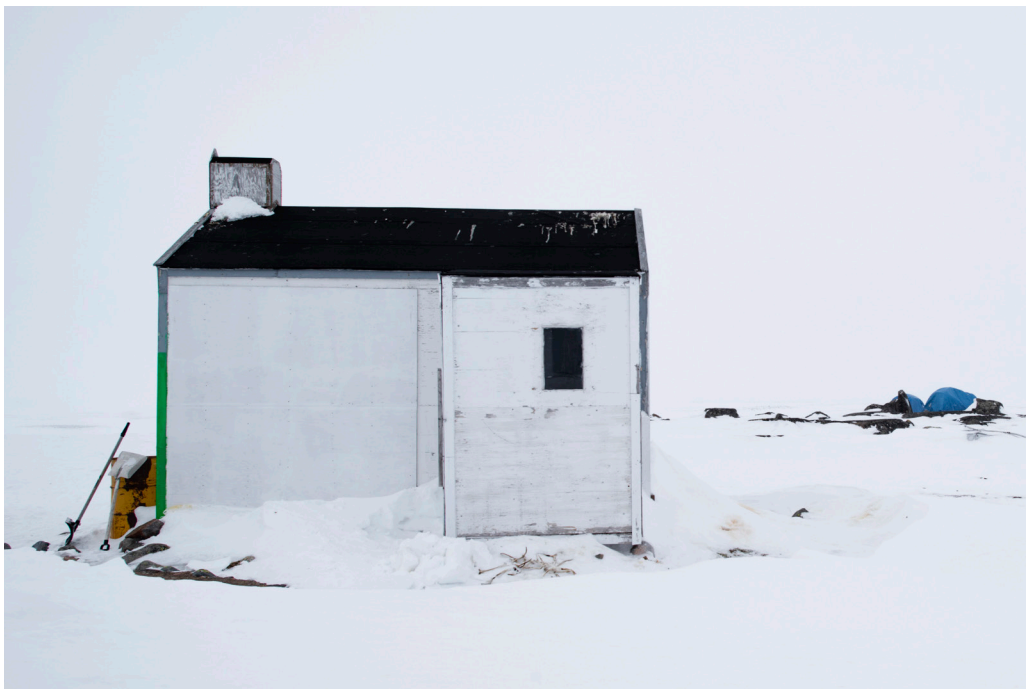
Fig.2.14 Bunkhouse from southwest (top) and east facade showing shower (below)
