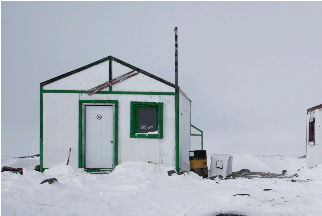
Fig.2.10 Equipment cabin west (top) and south (below) facades
