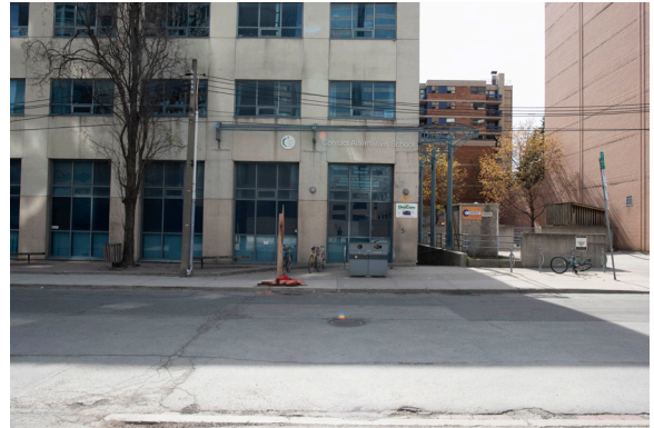
1 Existing school (Contact Alternative School)
