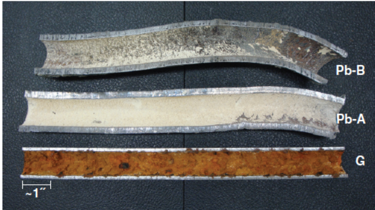
Figure 2.1 Internal corrosion scales of pipe samples that have been cut in half lengthwise. Pb (lead) segments Pb-A and Pb-B contain a fully uniform scale coating, while galvanized pipe G is tuberculated. Reprinted with permission from Scale Formation Under Blended Phosphate Treatment for a Utility With Lead Pipes (E467), by Wasserstrom, Miller, Triantafyllidou, DeSantis, and Schock, 2017. Journal – American Water Works Association. © 2017 American Water Works Association.
