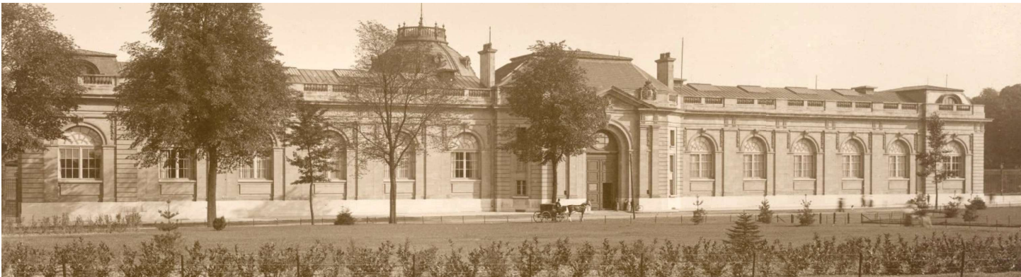
Fig 2.19 The Northern Face of the Royal Museum of Central Africa shortly after its construction.
