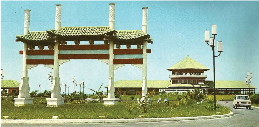
Fig 1.04 Mobutu's Pavillion in Nsele. As one of his favourite residences, it welcomed important visitors of state while Mobutu was in power. It was at this pavillion in Nsele that he declared the end of his one party rule. Upon the end of his reign and the reinstatement of a new presidential candidate, many of Mobutu's residences were looted and changed forever in what is referred to as the "pilage." The "pilage" was a week-long spree of looting and destruction in September of 1991 that was done by underpaid troops of the national army in major cities across the country resulting in hundreds of deaths. It had a horrible effect on the economy, ultimately turning military bases thriving markets for looted goods up for resale. This included his private residences and pavillions.
