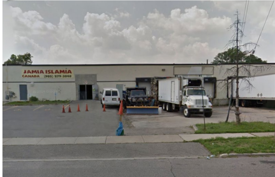
fig. 1 exterior of jamia islamia muslim centre and mosque, captured from Google street view
