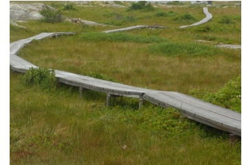
fig. 76 planks of wood are suspended over a landscape in Fogo Island, forming a light walkway that can be easily adapted to an uneven landscape
