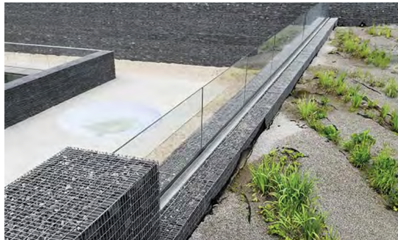
Figure 3.8: Part of the purification process is filtration through crushed granite as shown.
