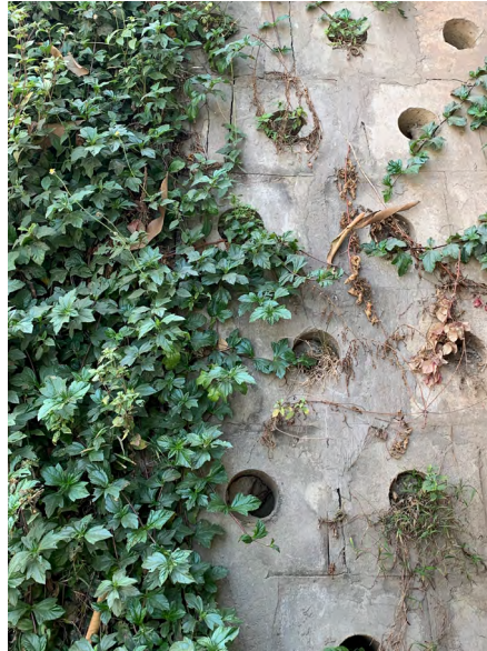
Figure 5.32: Close up of the concrete blocks supporting the slope.
