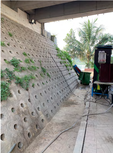
Figure 5.31: Concrete blocks line the wall. The openings through the concrete blocks allow greenery to grow.
