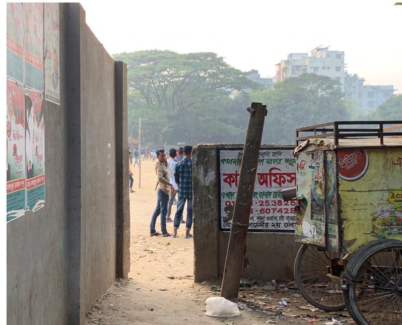
Figure 4.49: The wall around the T&T playground. Small gap remains for entrance.
