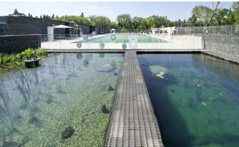
Figure 3.7: A panoramic photo showing the hydrobotanic pond where the filtration processes takes place.
