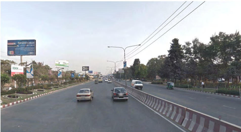
Figure 1.24: The central spine road running north south in the middle of Dhaka is part of the western embankment.
