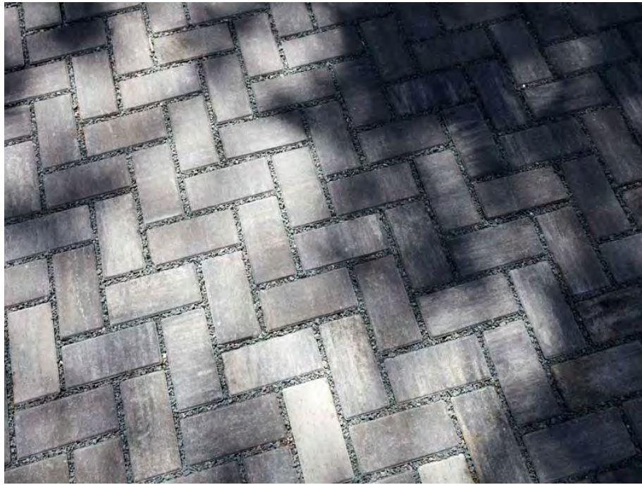
Figure 5.57: Permeable interlocking concrete pavers.
