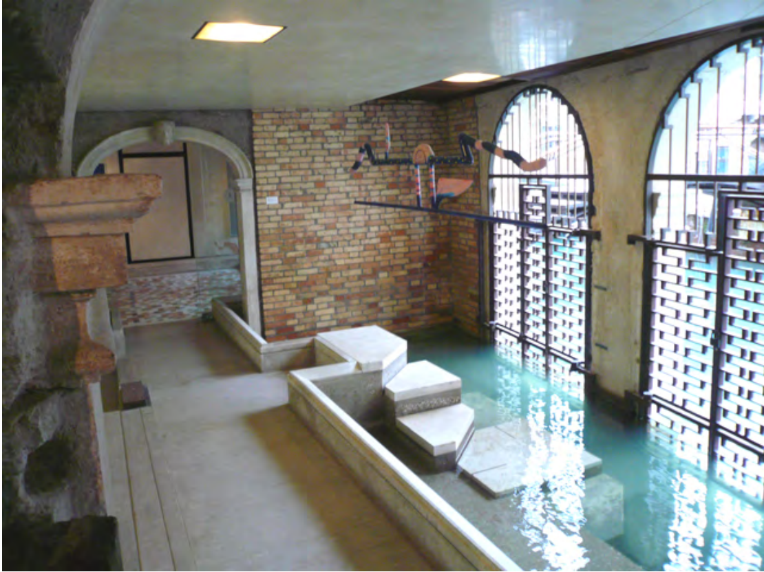
Figure 5.46: Carlo Scarpa's Palazzo Querini Stampalia in Venice. This building was designed to allow water into the building.
