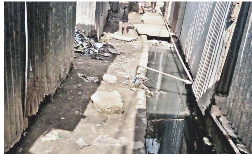
Figure 4.19: Unsanitary open drainage in the alleyways of the slum.
