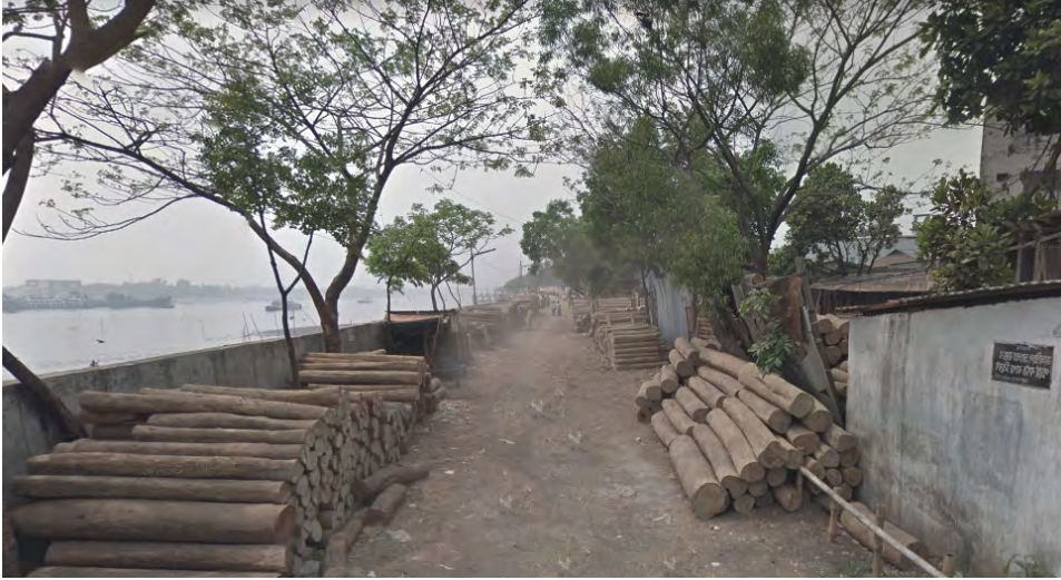
Figure 1.22: Flood wall constructed along Buriganga river to prevent the city from river flooding.
