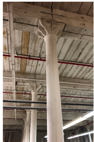
fig.3.62. Photograph of Existing Mill no.2 Decorative Capitals
