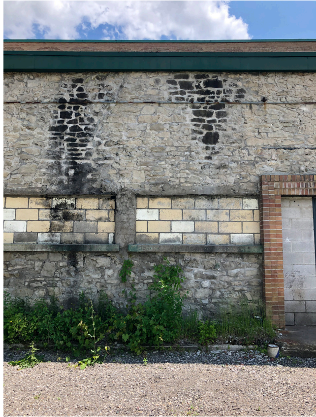
fig.3.52. Photograph of Collaged Facade
