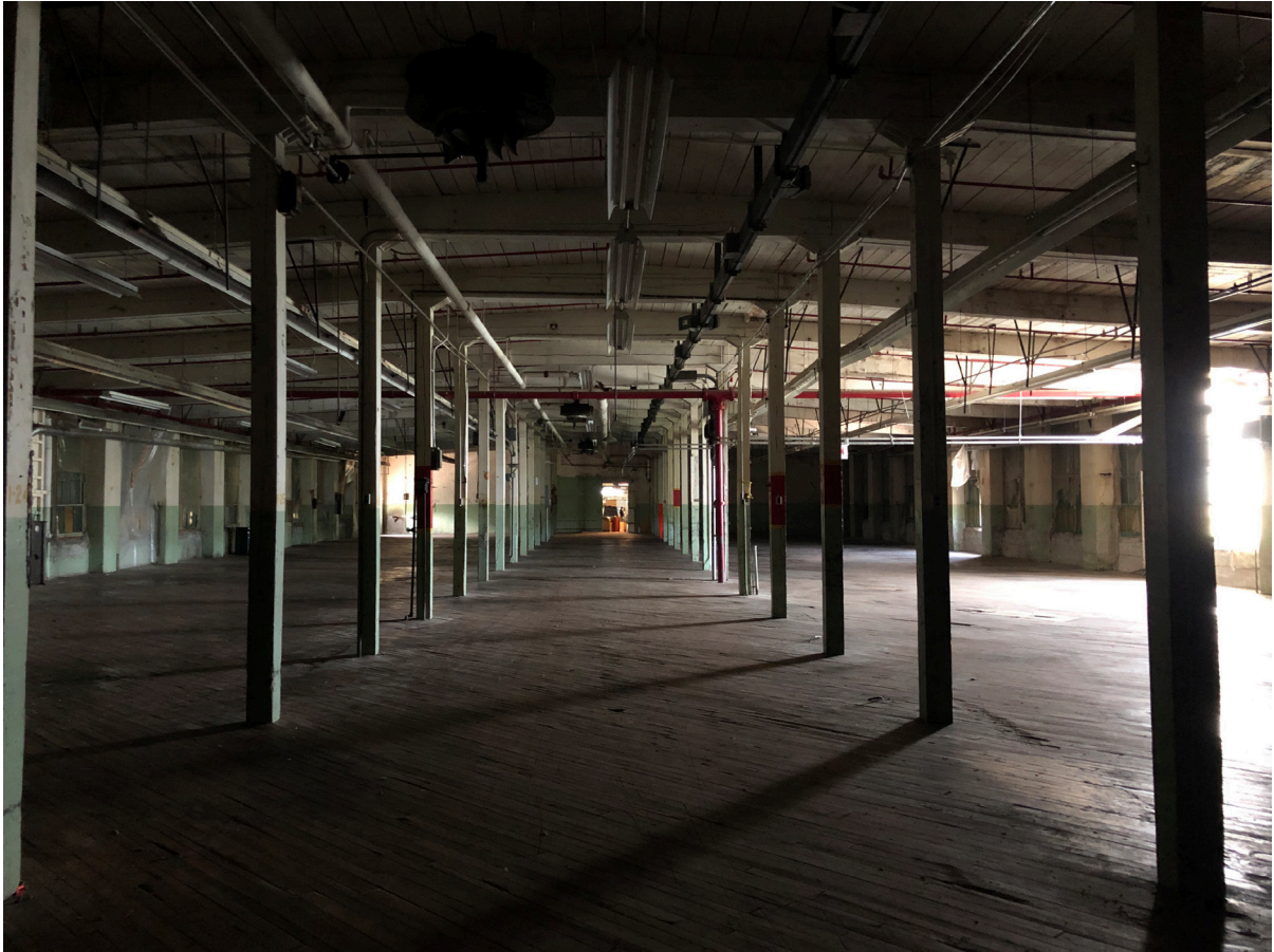
fig.5.15. Mill no. 3 Third Floor
