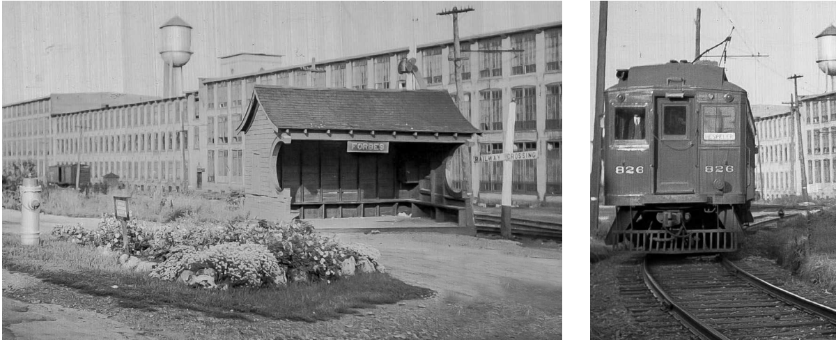
fig.3.49. Photographs of Train Stop and Rail Line at the Dominion Woolens & Worsted Factory
