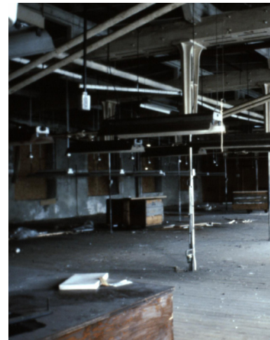
fig.3.43. Interior of Mill no. 1 Showing Queen Post Strut
