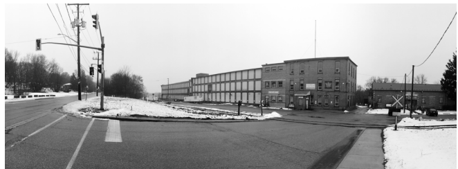
fig.3.21. Photograph of Building Today
