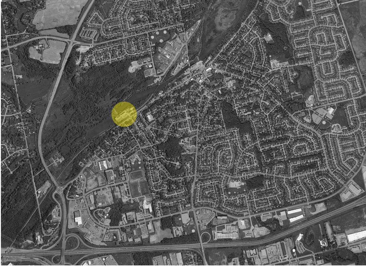
fig.3.7. Aerial Photograph of Hespeler, Ontario Site highlighted in yellow.
