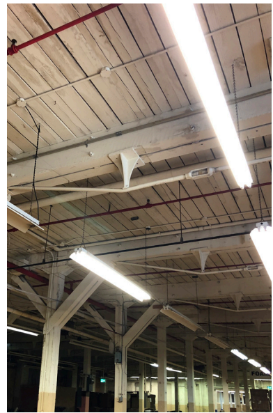
fig.3.58. Photograph of Existing Mill no.3 Queen Post strut
