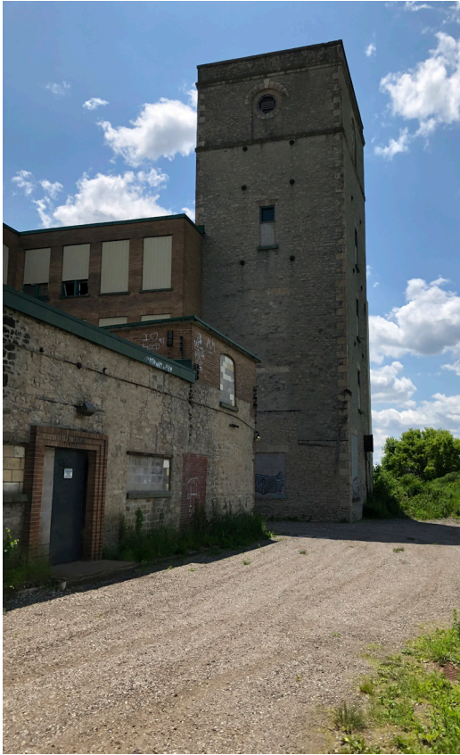
fig.3.51. Photograph of the Tower
