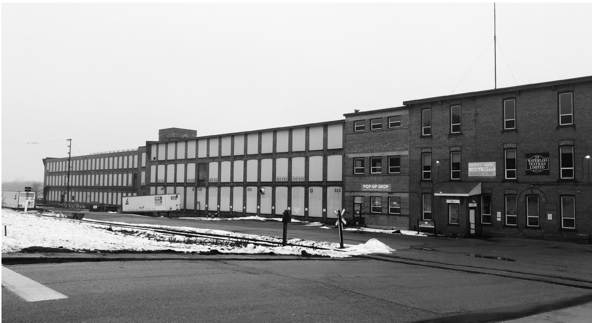
fig.3.8. Photograph of Existing Building on Site
