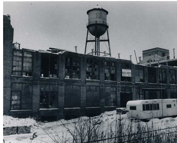
fig.3.17. Photograph of Partial Demolition
