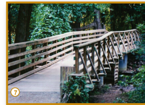
Bridge over Ellis Creek
