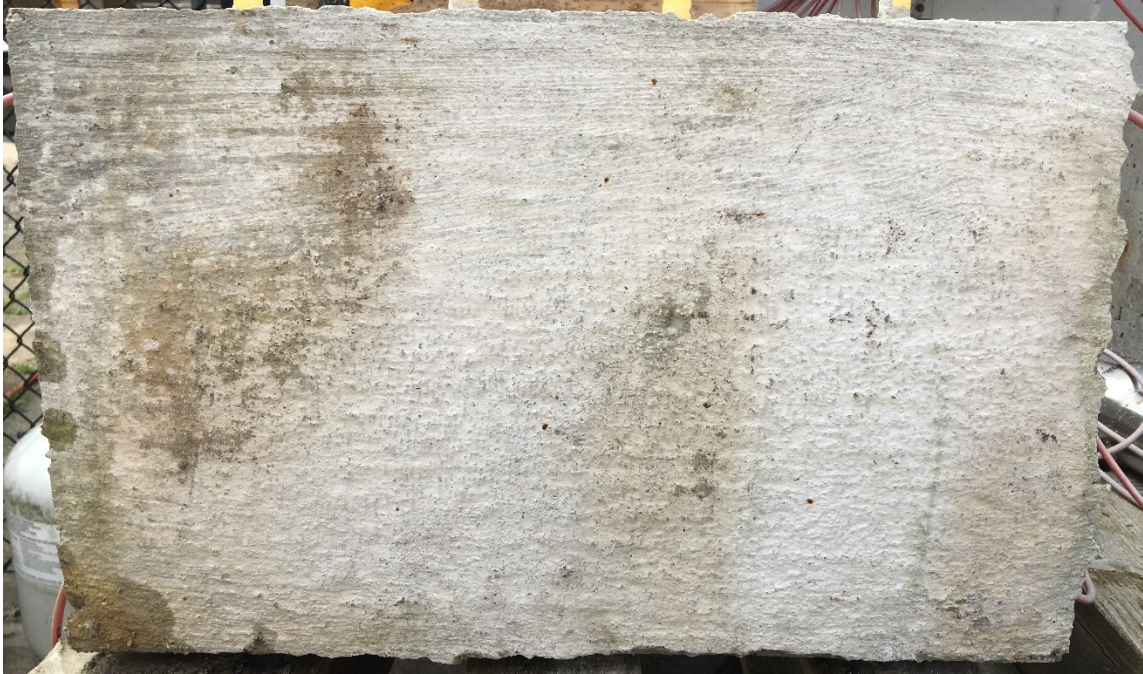
Figure 4-9: Bottom surface of outdoor specimen in Figure 4-8
