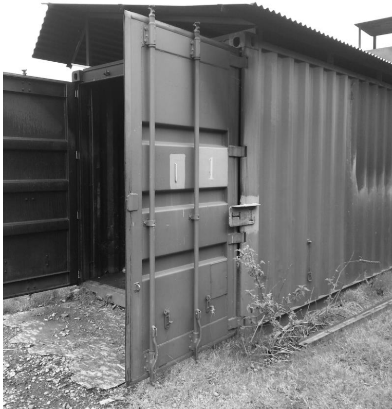
Figure 32: Roof (Dublin Fire Brigade)
