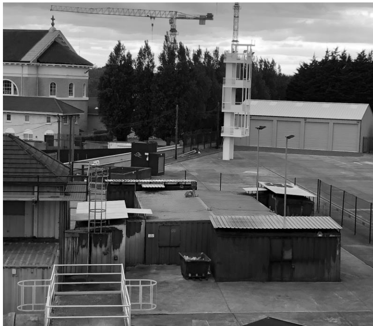
Figure 9: Dublin Fire Brigade Training Centre – reprinted with permission from [45]
