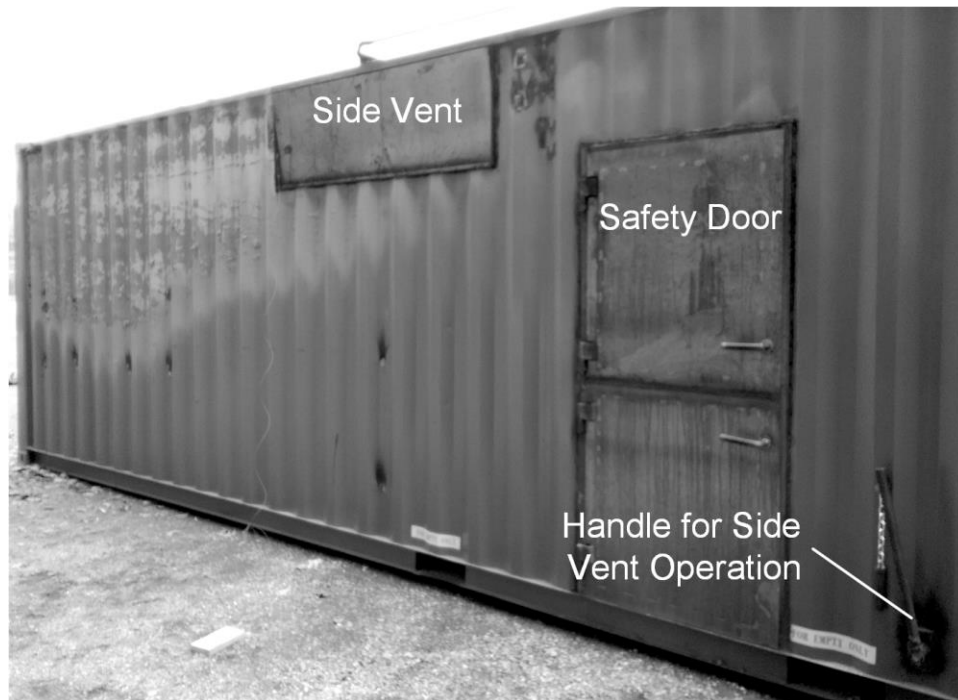
Figure 24: Side vent and safety door
