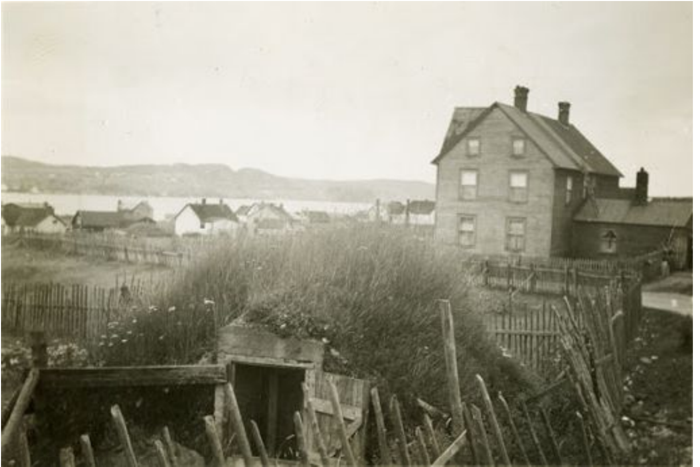
Figure 1.2 Twillingate Home and Root Cellar
