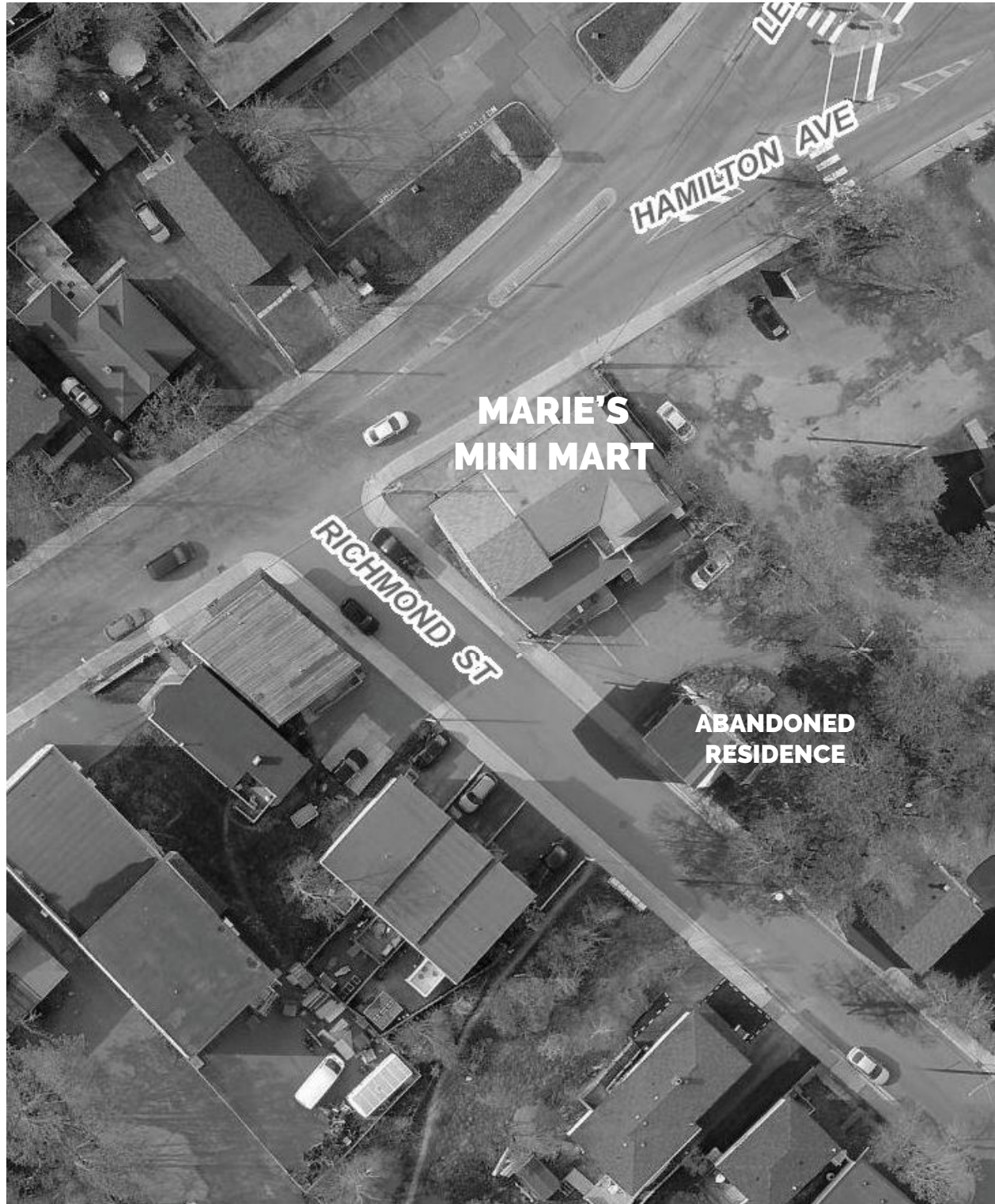
Figure 4.3 Aerial view of Marie's Mini Mart and surrounding neighbours.
